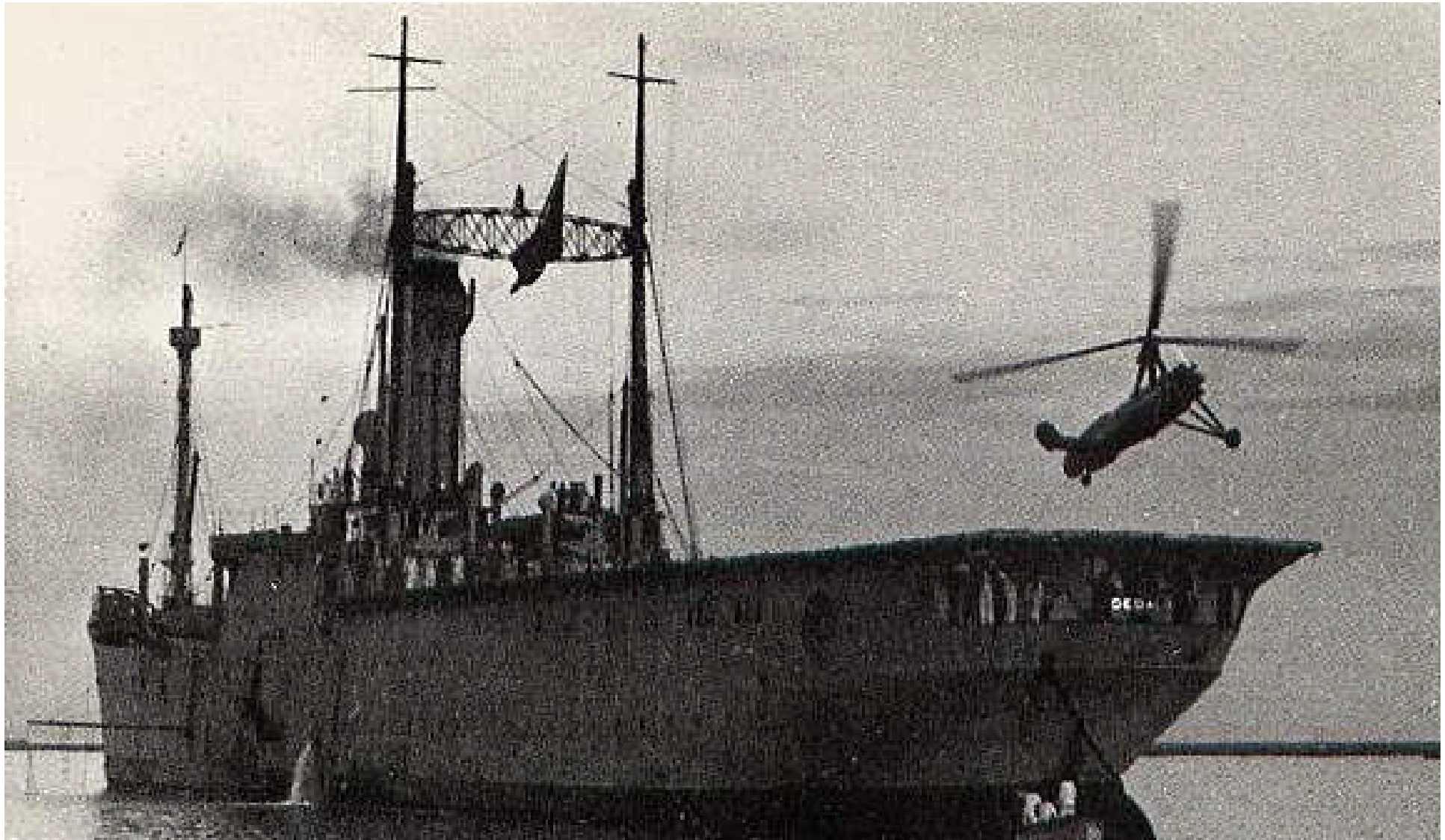
Above: on March 7 th 1934, a Cierva C.30 Autogiro piloted by Juan de la Cierva became the first rotary wing aircraft to take-off and land on the deck of a ship when it performed trials on board the Spanish Navy Seaplane Tender Dedalo
