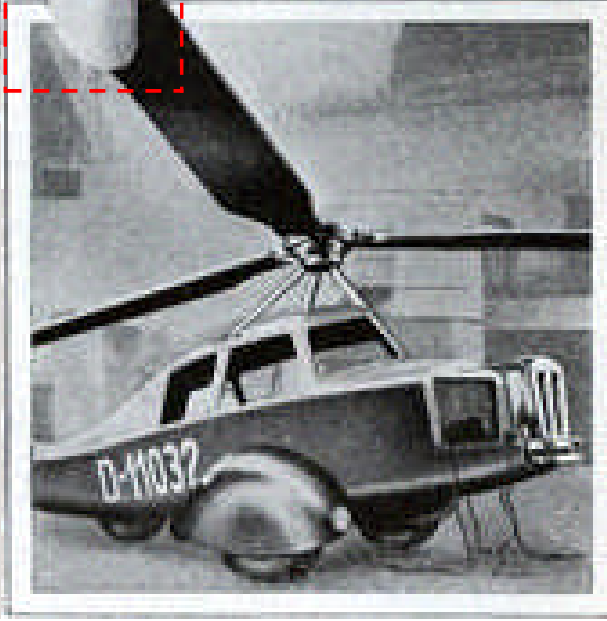
Above: caption: "Artist's drawing shows the 'flying auto' doing duty as both plane and auto. When it is to negotiate the highways the gyro blades are disengaged and power applied to the wheels." Right: caption: "Motor is mounted in the front as in an auto, the power being transmitted from there to either the gyro blades or the front wheels. Forward propulsion of the plane is obtained through action of the little vertical fins on the gyro blades."
