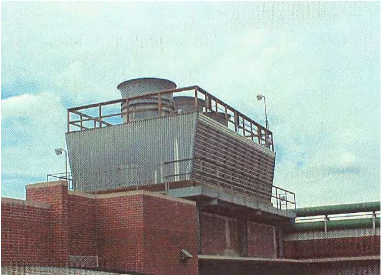
Figure 7 Cross-flow cooling tower
