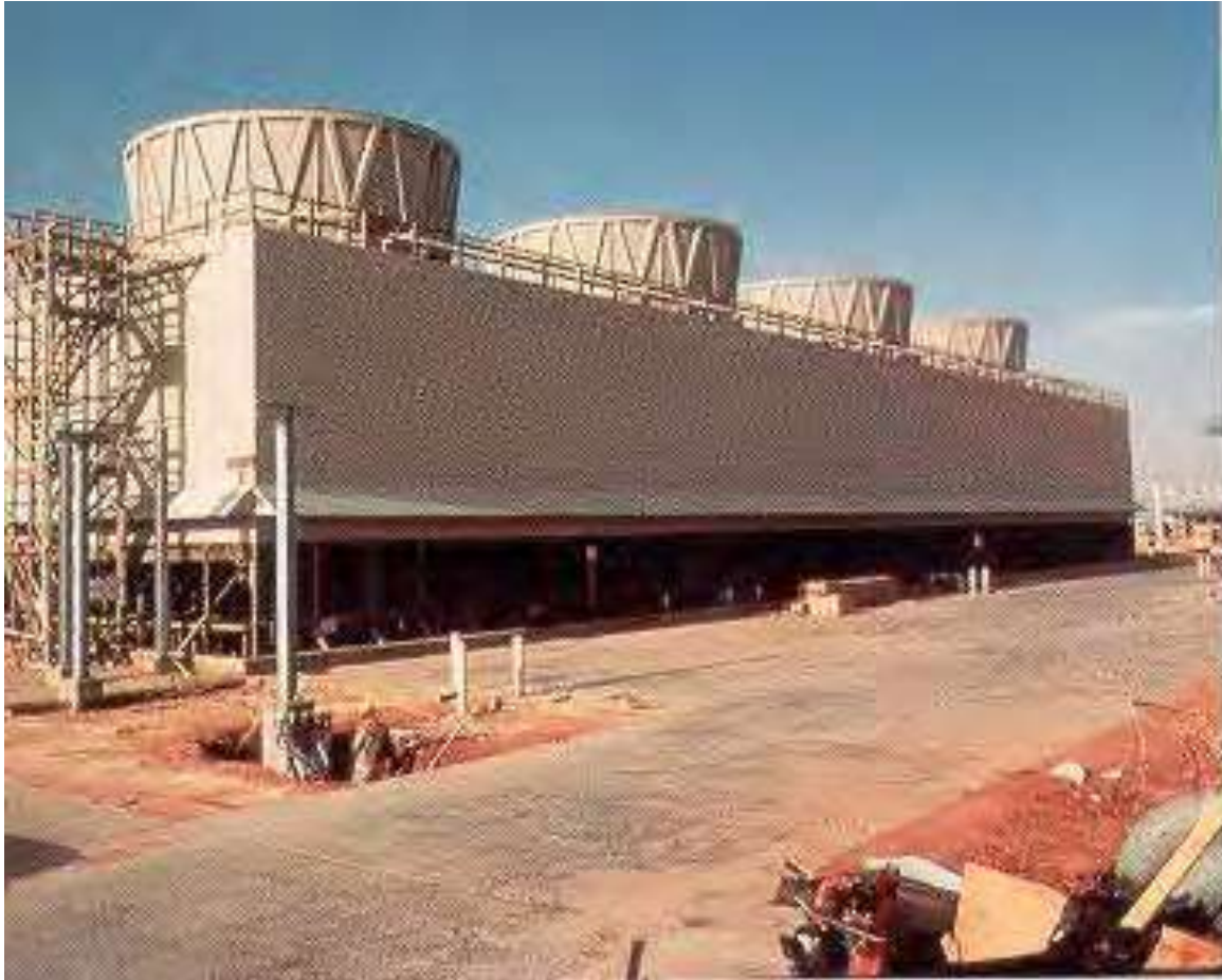
Figure 9 Counter-flow cooling tower
