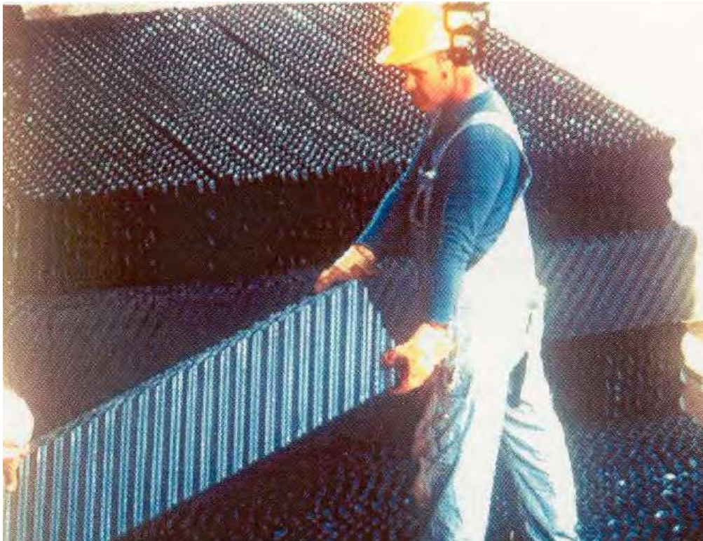
Figure 11 High-efficiency cooling tower film fill
