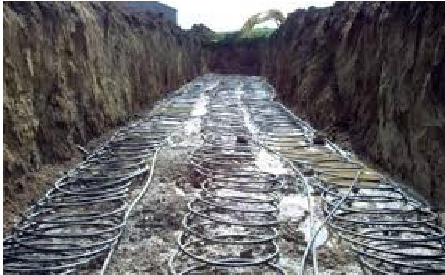
Figure 5. Single “slinky” pipe system
