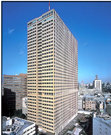
Left: in April 1968, Nippon-Otis completed installation of thirty-five elevators and eight escalators in what was to become Japan’s first skyscraper; the 512-foot Kasumigaseki Building in Tokyo. The Otis units included nine elevators with a speed of 1K fpm (considered the most advanced elevators at the time of their installation). The thirty-six floor Kasumigaseki Building was the first modern high-rise building in post-WWII Japan. 983
