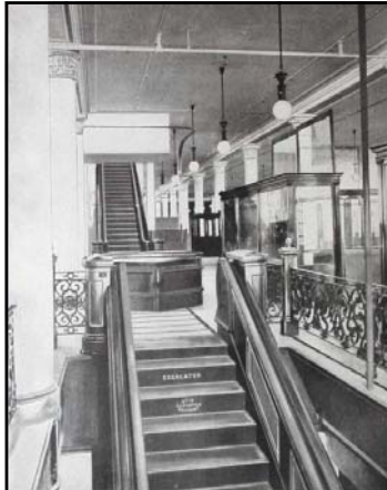
Left: caption: "Escalators in the store of Messrs. R.H. Macy & Co., New York, showing the upper landing of the first Escalator and the second Escalator in the background. The ample space allowed in which to step from the Escalator is clearly shown, and the moving hand rails and the shunt may also be seen. The Escalators serving the upper floors are located above."
