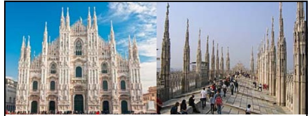
Above L&R: the Cathedral of Milan has 135 spires and, in one of them, an Otis elevator. What began in 1997 as an Otis modernization project in preparation for the Vatican's 2000 Jubilee became a new prestige elevator, installed inside a spire of Italy's largest and most intricate example of Gothic Architecture (the new elevator replaced an Otis unit installed in 1961). It's used primarily to take visitors to the cathedral's roof for a fantastic view of the city through a forest of spires and 2,245 white marble statues.
