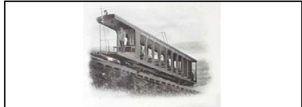
"...The Mt. Beacon Incline Railway was built by this company. The length of this road is 2,200 feet, with a rise of 1,200 feet. The average grade is 64 per cent. The speed of each car is 500 feet per minute and the seating capacity 54 persons. Each car is equipped with the Otis double-grip safety device. The Otis Electric Hoisting Engine for operating these cars is provided with two 75-horse-power electric motors controlled by the Otis electric switch and magnet system..." RE: excerpt from an Otis Elevator Company brochure (ca. 1905) 704 Above: caption: "Mt. Beacon Incline Railway Car"
