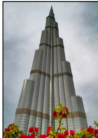
The Burj Khalifa (left) opened on January 4 th 2010. It's 828-meters to the top of the spire (2,717-feet), and has 162 floors. The mega-skyscraper was designed by Adrian Smith of the architectural firm Skidmore, Owings & Merrill and constructed by South Korea's Samsung Corporation ( Turner Construction International served as Construction Manager). The mixed-use building features offices, 1,044 residential apartments (including 144 Armani Residences ) and 160 ultra-luxury hotel rooms at the Armani Hotel Dubai . The Corporate Suites comprise 49 floors. Initially, it was called "Burj Dubai," but the name was changed just before completion to honor Sheikh Khalifa of Abu Dhabi - the president of the United Arab Emirates (in 2009, he borrowed money to complete the building when Dubai had severe financial difficulties)
