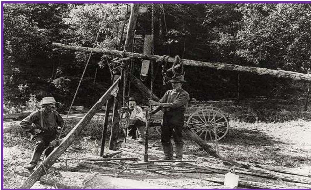
John Grandin used a spring-pole to drill deeper than the famous Drake well of 1859
