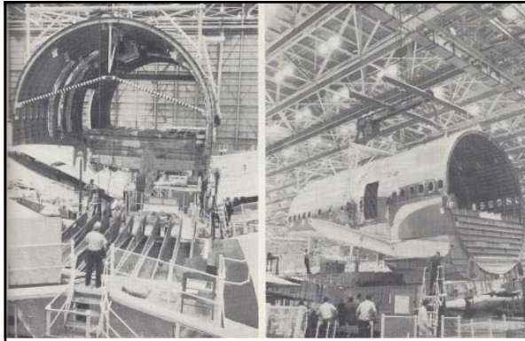
Above L&R: caption: "Wing-fuselage mating has been simplified by using only a short fuselage section. Section 44 is placed atop the wing carry-through section and bolted in place (left). Landing gear support is I-beam extending from fuselage (right)." 447
