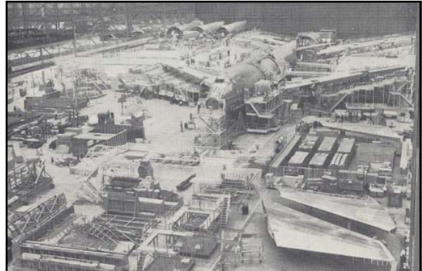
Above: caption: "Final body join position, where three major sections are fastened together, is located forward of the wing-stub join area. Landing gear and tail also are installed here." 448
