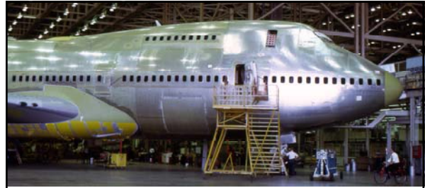
At the time of its completion in 1968, the original Boeing 747 factory at Everett - measuring 42.8 acres (1.9 million square-feet) and 205.6 million cubic-feet in volume, instantly became the world's largest building. Remarkably, the factory was so capacious, it began generating its own weather systems. A then state-of-the-art circulation system had to be installed because clouds (the product of accumulated warm air and moisture) were forming inside. Then as now, there is no climate control system for temperature. In the winter, machinery, body heat and residual heat from lights keep it warm while in the summer, the doors are opened to cool the building.
