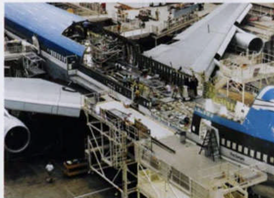
D. Structural preparation.
