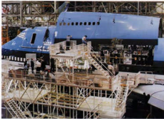
A. Existing U/D crown removed.
