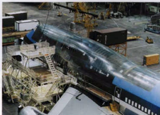
F. New structure in place.
