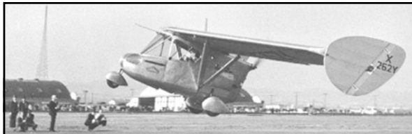
Above & Left: caption: "The 1937 Waterman Arrowbile ." Waldo Waterman modified a six-cylinder upright, 100-hp Studebaker engine to build this flying car in 1937 (it carried two people). Only three Arrowbiles (a/k/a Arrowplane ) were ever produced, though Waterman later attempted to produce roadable versions in the 1940/50s. 405
