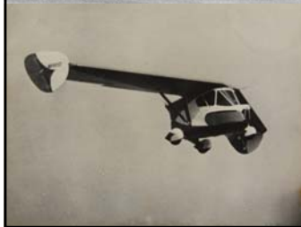
Above & Left: caption: "The 1937 Waterman Arrowbile ." Waldo Waterman modified a six-cylinder upright, 100-hp Studebaker engine to build this flying car in 1937 (it carried two people). Only three Arrowbiles (a/k/a Arrowplane ) were ever produced, though Waterman later attempted to produce roadable versions in the 1940/50s. 405
