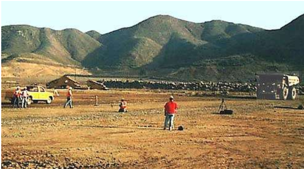
Figure 5: This photo shows the 60-ton construction loader (right) and the yellow pick-up truck (left) at their initial respective position. The message the contractor wanted to deliver was that the driver of the loader is seated so high above the ground that he will not see the pick-up truck. In addition, the loader is so massive and heavy when fully loaded that the driver would not even feel his collision with the pick-up truck.
