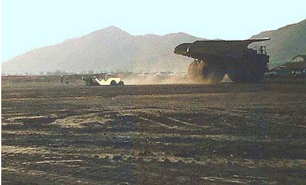
Figure 6: This photo shows the 60-ton construction loader proceeding on its course without deflection after flattening the pick-up truck (yellow heap, left of center). The contractor wanted to impress his staff and convince them to stay away from the construction loaders in order to avoid the possibility of an accidental encounter. It is evident in this case that the contractor did not spare any expense in delivering his message. His derived benefit came from a sensitized work force to this particular hazard on the work site.
