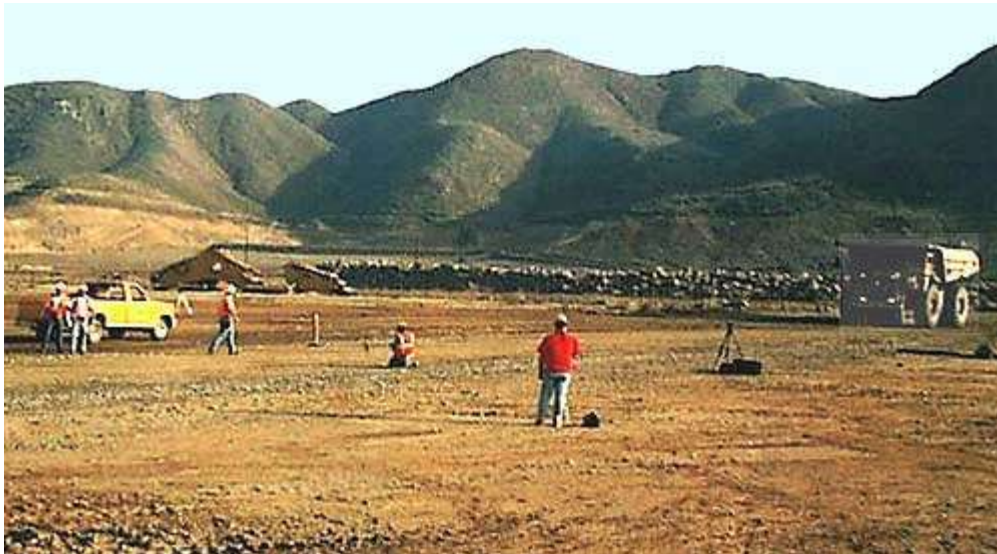
Figure 5: This photo shows the 60-ton construction loader (right) and the yellow pick-up truck (left) at their initial respective position. The message the contractor wanted to deliver was that the driver of the loader is seated so high above the ground that he will not see the pick-up truck. In addition, the loader is so massive and heavy when fully loaded that the driver would not even feel his collision with the pick-up truck.
