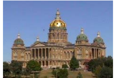
Iowa Capitol Building
