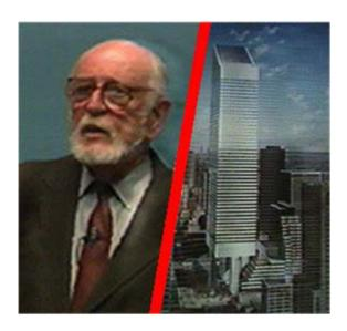
Half the gravity and all the wind loading is through the trussed frame on the outside of the building with the core carrying the remaining gravity loads. LeMessurier used a diagonal bracing design transferring weight to the columns and added a tuned mass damper to reduce wind sway of the building. The tuned mass damper consisted of a 400-ton concrete block that counteracts swaying.
