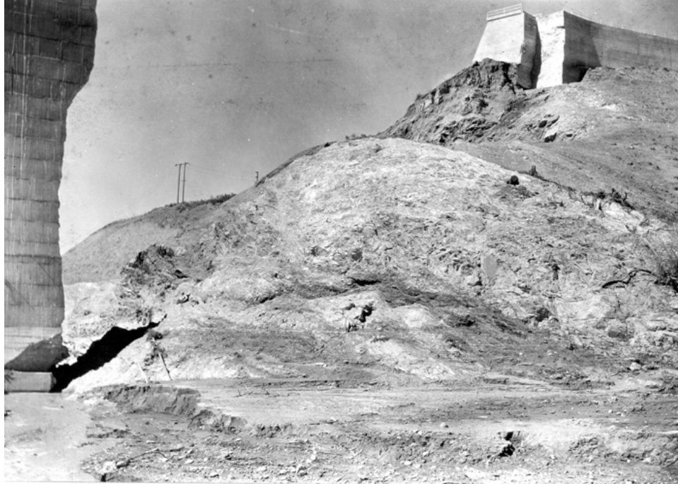
St. Francis Dam, Former West Abutment (Attribution: U.S. Geological Survey Photographic Library) Figure 6
