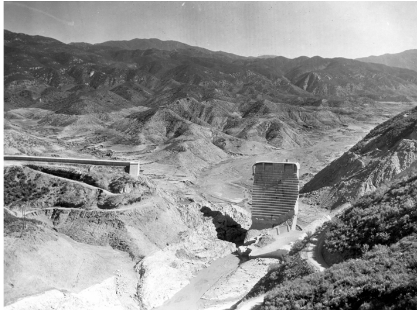
St. Francis Dam, March 17, 1928 (Attribution: U.S. Geological Survey Photographic Library)
