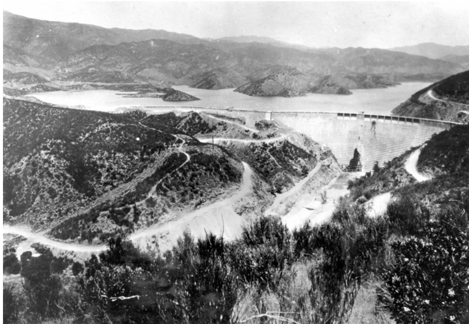
St. Francis Dam
