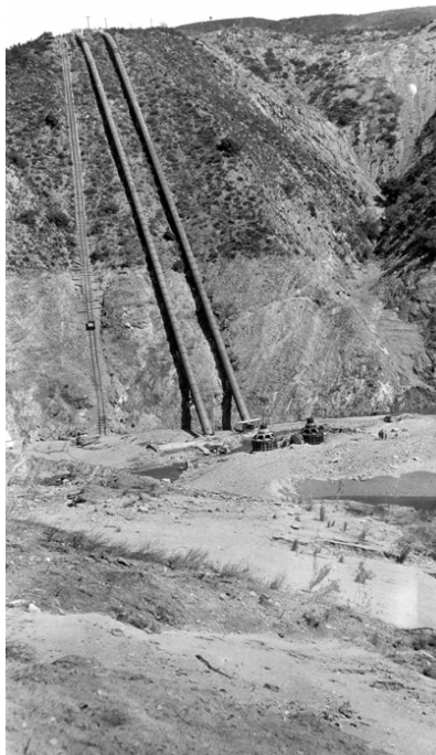
Remains of downstream powerhouse (Attribution: U.S. Geological Survey Photographic Library) Figure 7
