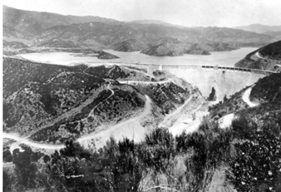
St. Francis Dam (Attribution: U.S. Geological Survey Photographic Library)
