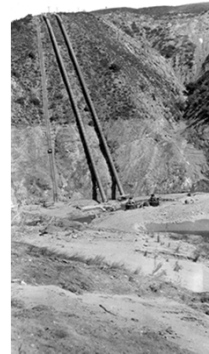
Remains of downstream powerhouse (Attribution: U.S. Geological Survey Photographic Library)
