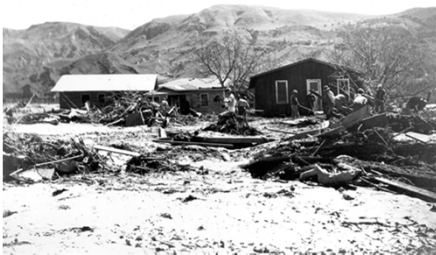
Flood damage at Santa Paula (Attribution: U.S. Geological Survey Photographic Library)
