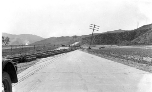
Dislocated railroad tracks (Attribution: U.S. Geological Survey Photographic Library)
