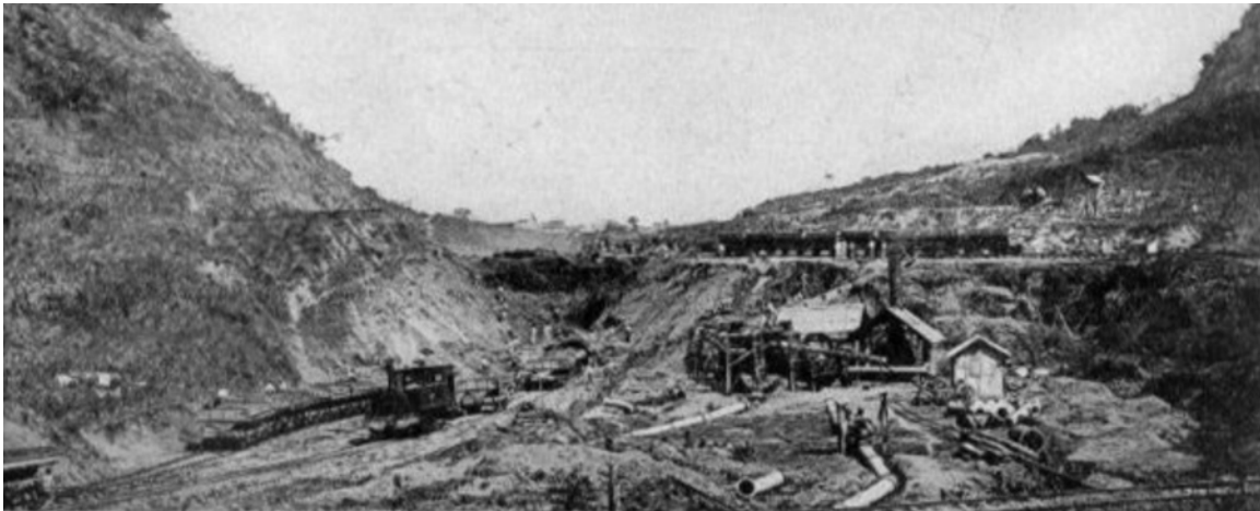
Figure 1 French canal excavation work at Cucaracha, 1885
