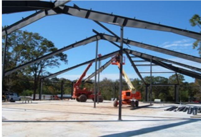
Tapered Beam Source: Timeline Builders
