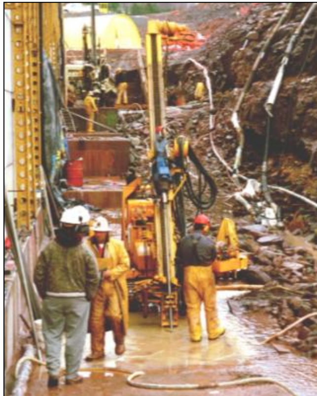
Figure 13-20. Drilling operations concurrent with RCC dam construction.
