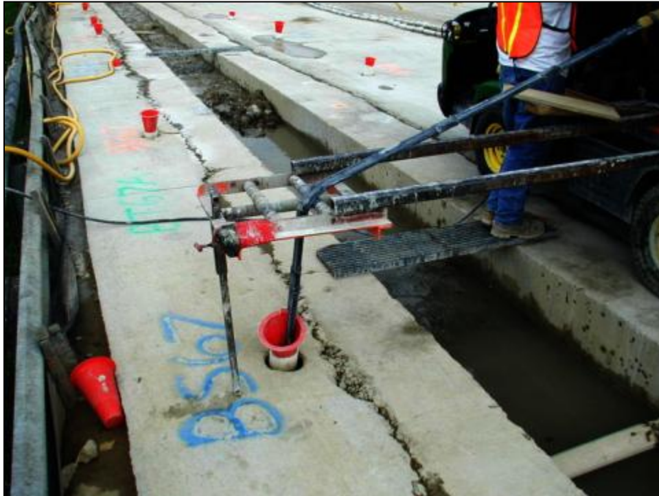
Figure 15-3. Typical numbering and color-coded marking scheme for grout holes.
