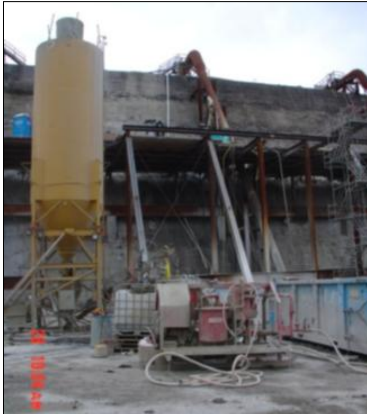
Figure 23-8. Typical grout batching plant being fed by bulk cement from a silo at Gilboa Dam, NY.
