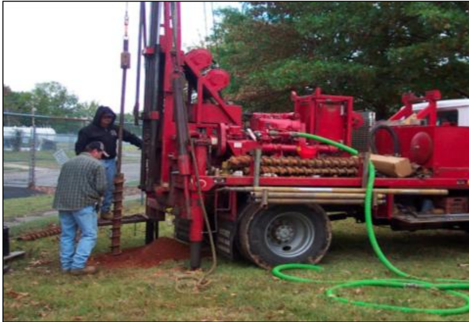
Figure 8-2. Hollow stem auger system in use.
