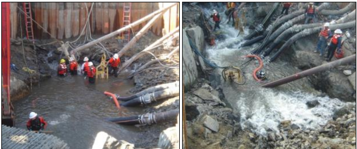
(Courtesy of Cianbro and Colonial Pipeline Company)
