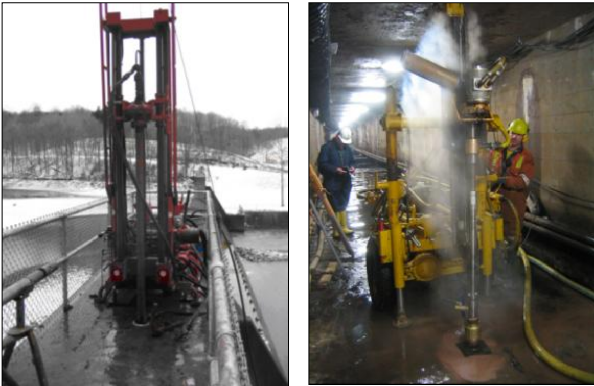
Figure 9-3. Track-mounted and hand-held high-speed rotary drills.
