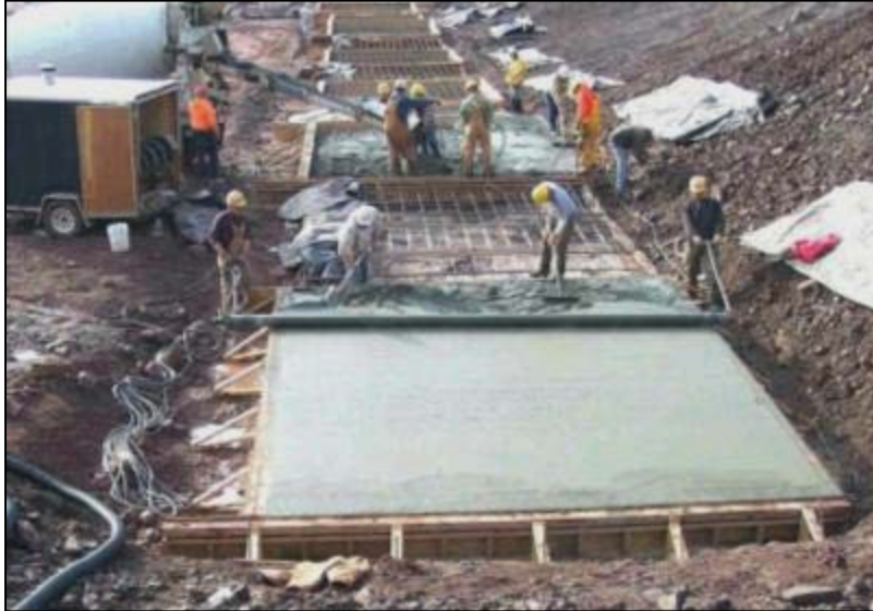
Figure 13-18. Grout cap used on a smooth, slaking rock surface.
