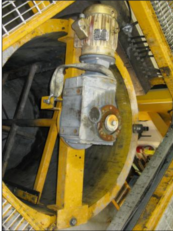
(Courtesy of Advanced Construction Technique.)
