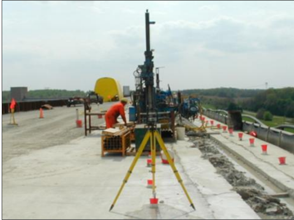
Figure 9-1. Use of conventional survey equipment to align a drill rig.
