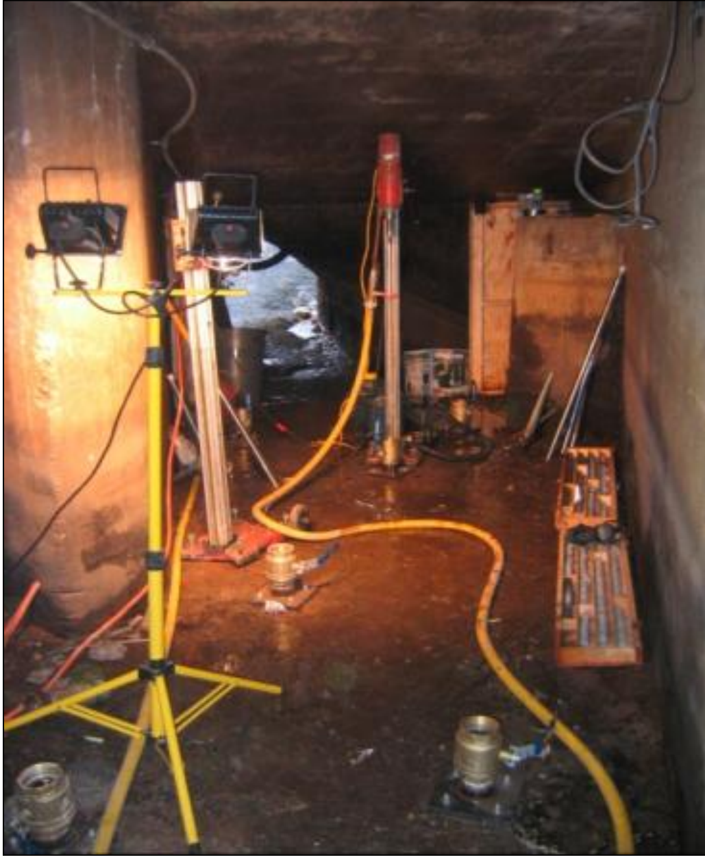
Figure 22-5. Grout holes for injection of HMG to fill a void beneath conduit.
