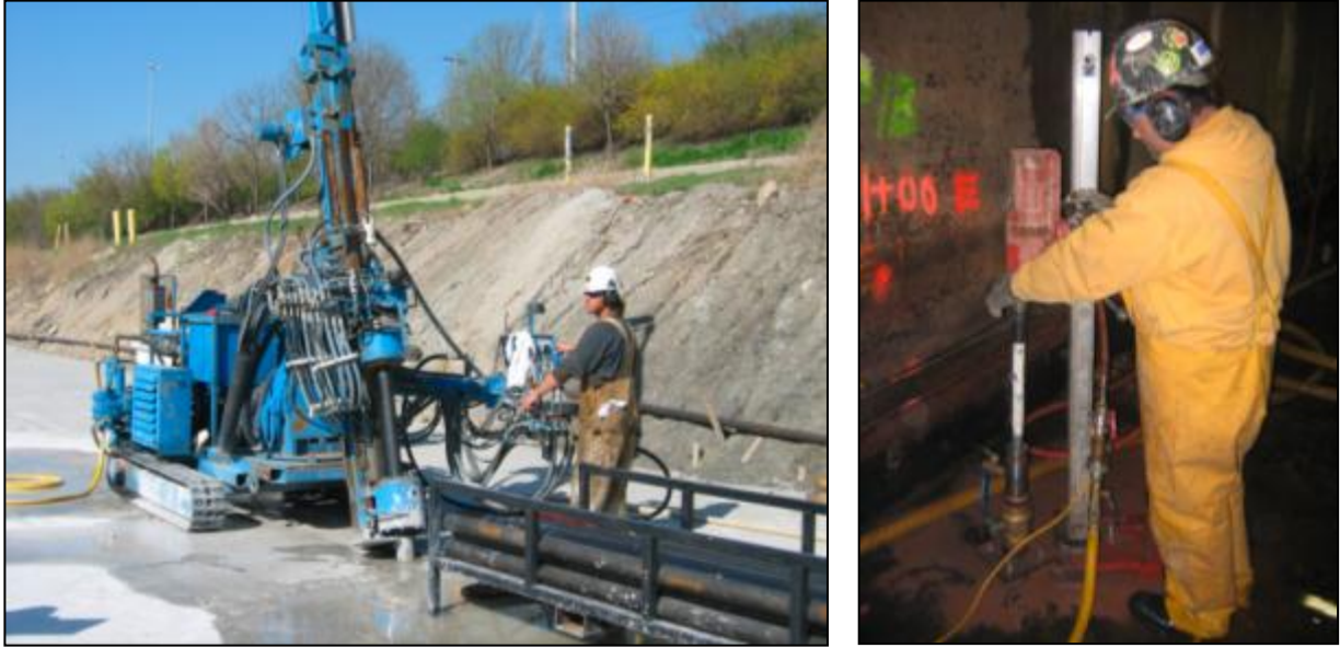
Figure 9-3. Track-mounted and hand-held high-speed rotary drills.
