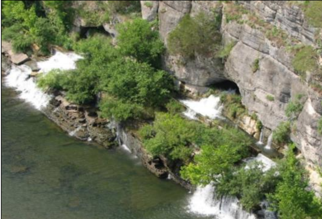
Figure 17-19. Elliptical tube cave features at Center Hill Dam (Nashville District).
