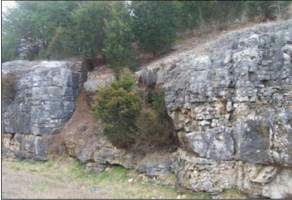
Figure 4-16. Limestone with solution features, varied bed thickness, and vertical joints at a highway rock cut in south central Kentucky.
