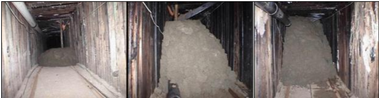
Figure 22-3. Time-lapse photos showing the advancement of LMG injected into a tunnel.
