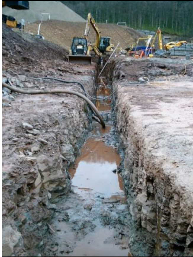
Figure 13-15. Heavily jointed rock suitable for excavating a cutoff cap.
