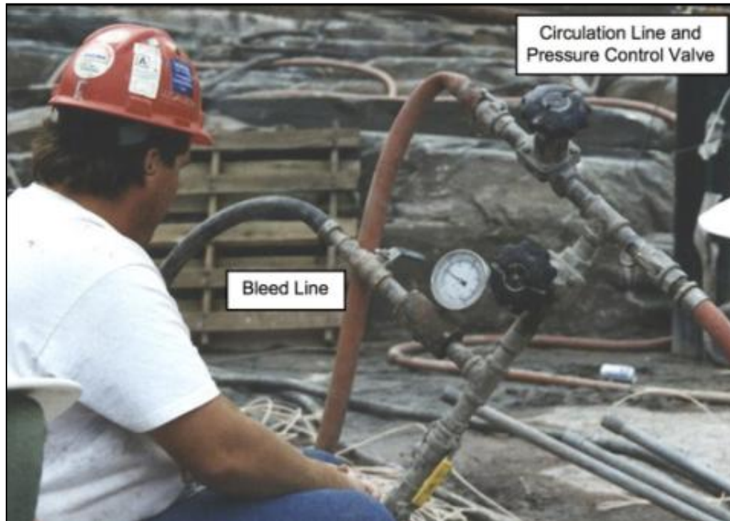
Figure 15-24. Standpipe arrangement for unstable grouts equipped with a bleed valve.
