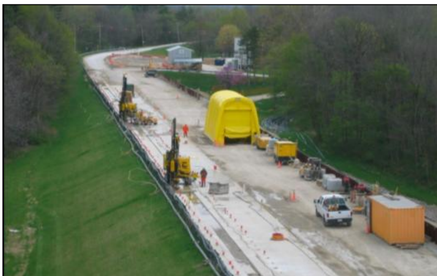
Figure 19-4. Pre-grouting for the Mississinewa Dam cutoff wall.
