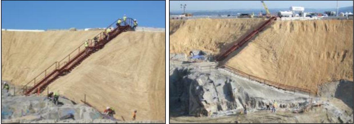
Figure 13-30. Typical access stairways on abutment areas, Folsom Dam (Sacramento District).
