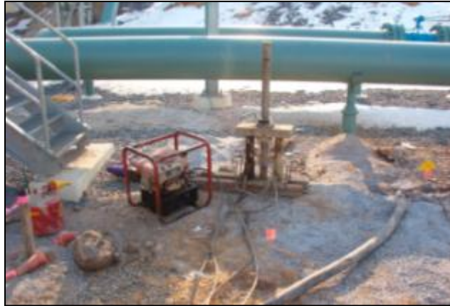
Figure 27-6. Casing withdrawal using extraction jacks.
