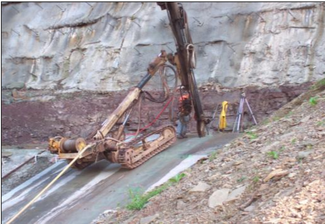
Figure 9-6. Air-track, top-hole percussion drill.
