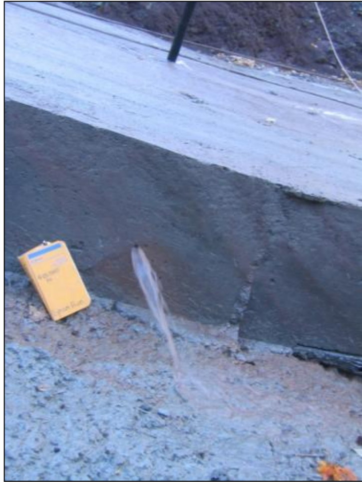
Figure 13-10. Porous grout cap requiring chemical grouting.
