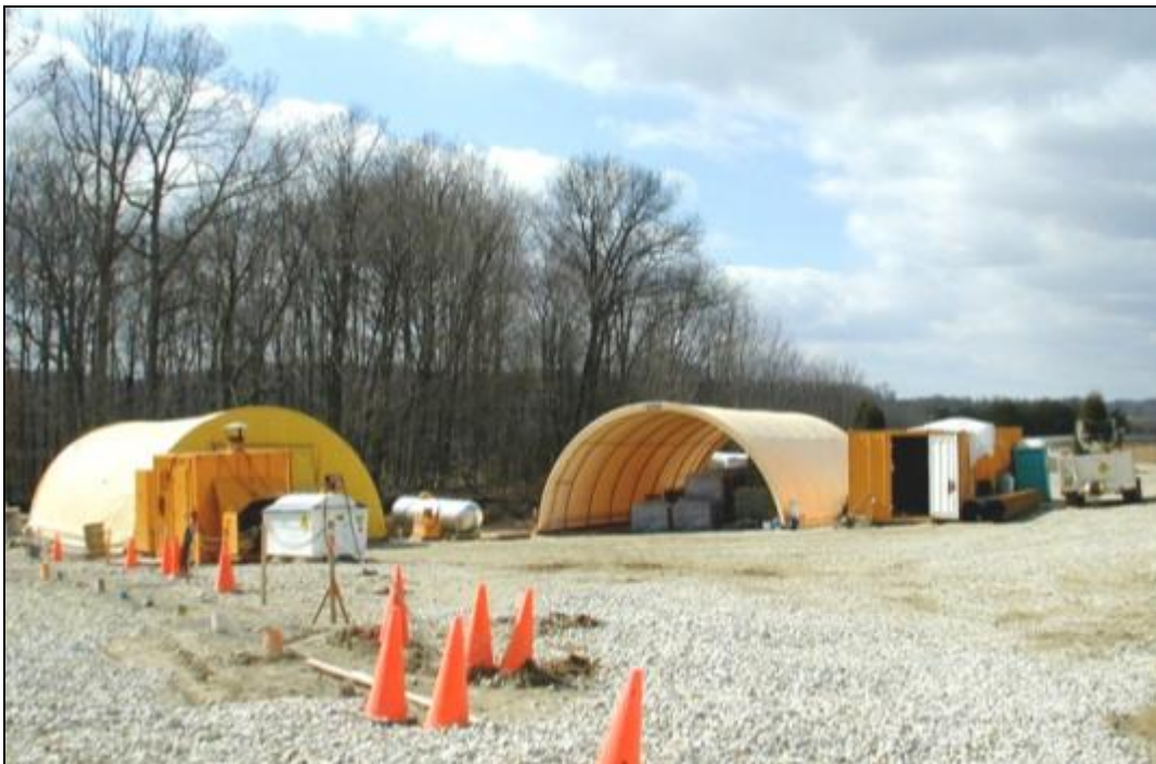
Figure 13-35. Winter-ready site with covered equipment storage, a fully enclosed and heated shelter for materials and mixing plant, and a water heating system.
