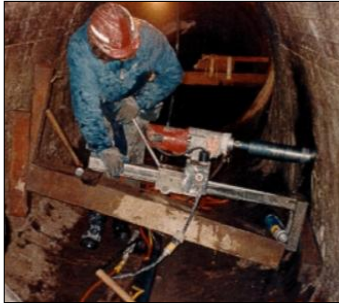
Figure 21-4. Drilling a grout hole inside a conduit
