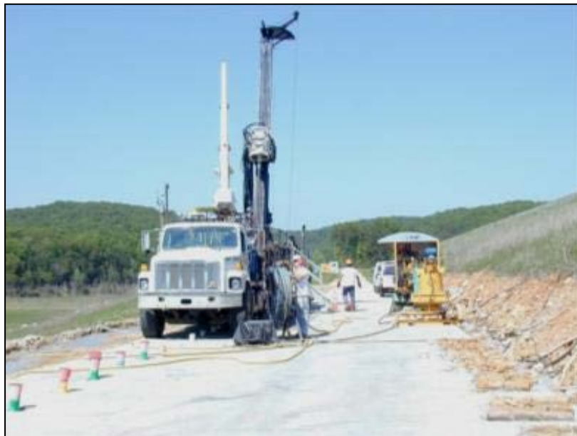
Figure 13-31. Hard surface platform with a cross slope leading to a collection trench.
