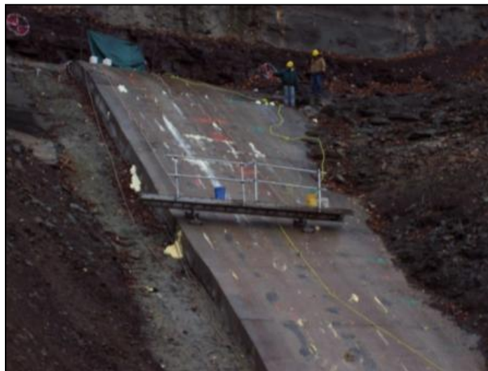
Figure 7-8. Urethane grouting used to waterproof the grout cap.
