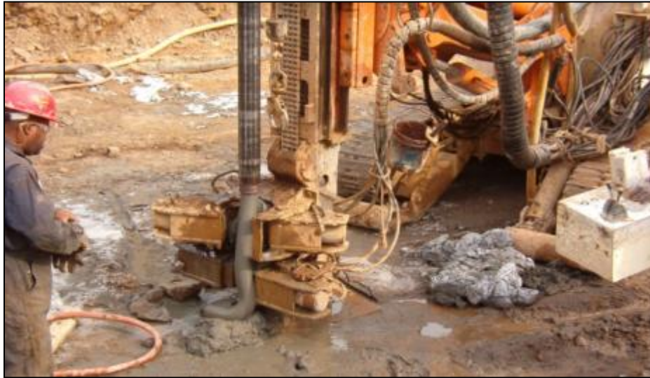
Figure 27-4. Stiff mortar-like compaction grout material being extruded through casing.
