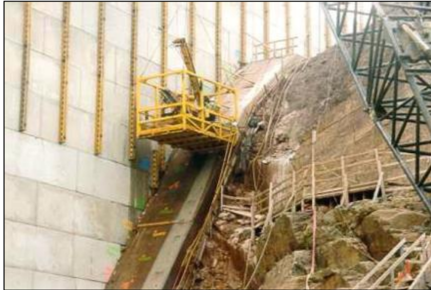
Figure 13-13. Crane-supported drilling platform on a steep abutment.
