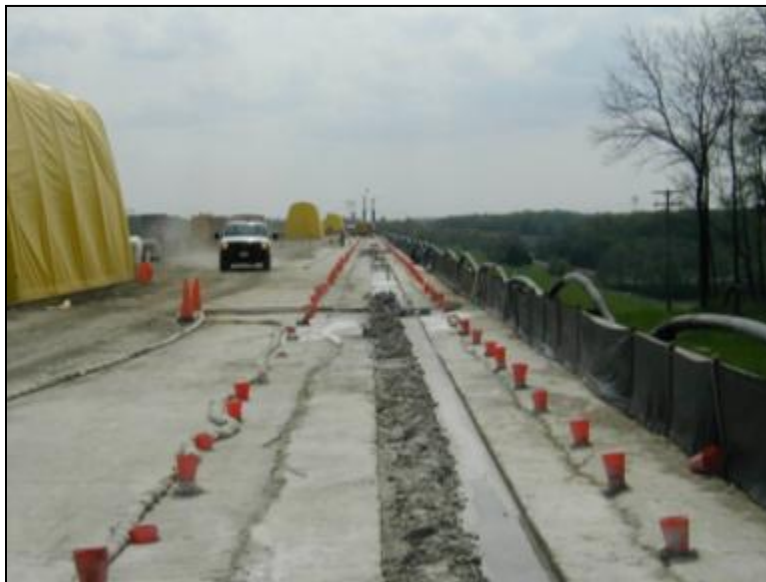
Figure 13-2. Hard surface platform after extensive drilling and grouting operations.
