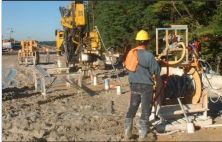
Figure 13-1. Gravel drilling and grouting platform after a short period of use.
