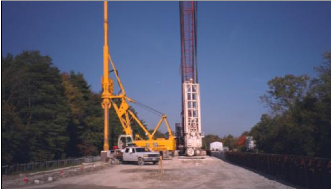
Figure 19-1. Hydraulic clamshell and hydromill machines at Mississinewa Dam (Louisville District).
