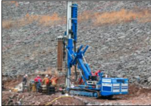
Figure 8-8. Duplex drill installing relief wells at the toe of a dam.
