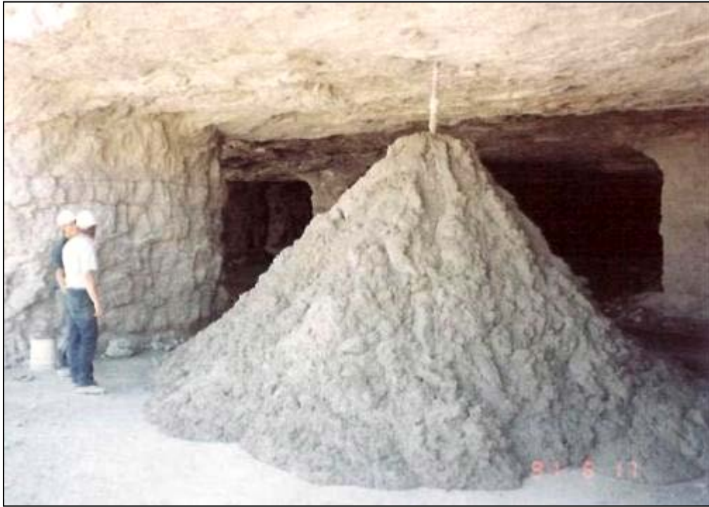
Figure 22-2. LMG injection into a mine void.
