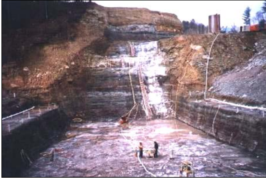
Figure 13-7. Smooth valley and abutment surfaces in sedimentary rock sufficiently soft to permit significant smoothing by excavation.
