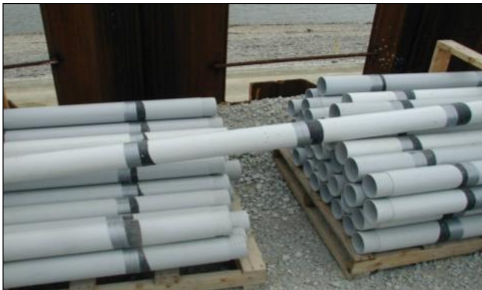
Figure 17-44. Sleeve-port casing to be installed in overburden and soil-filled dissolution features at Mississinewa Dam in Indiana (Louisville District).
