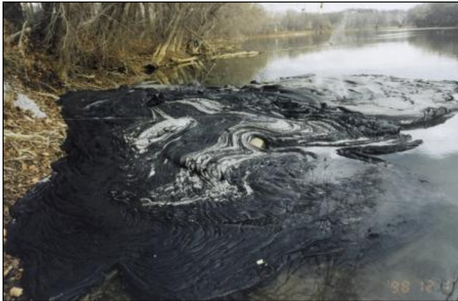
Figure 7-3. Hot bitumen and HMG from co-injection that escaped to the surface from deep karst.
