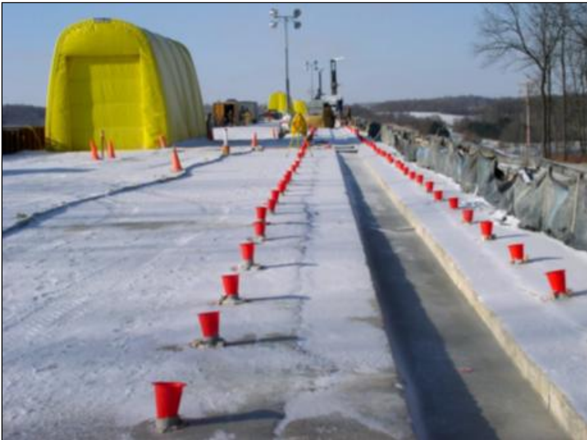
Figure 19-5. Pre-grouting lines for the Mississinewa Dam cutoff wall (Louisville District).
