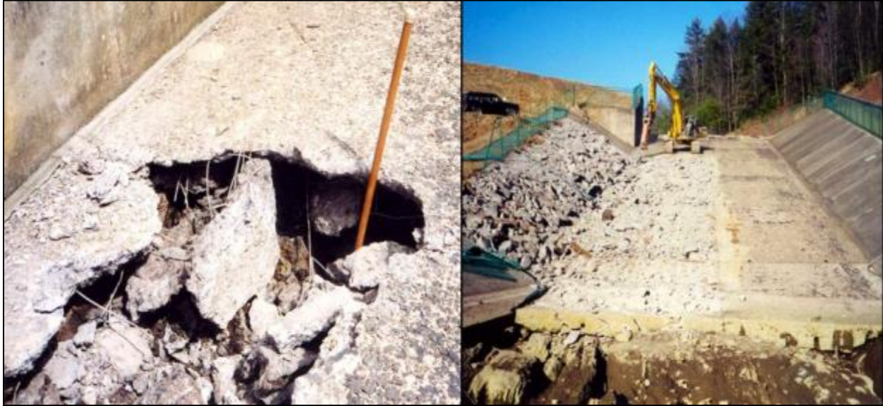
Figure 22-4. Extensive network of large voids beneath a spillway slab, which necessitated demolition and construction of new spillway.
