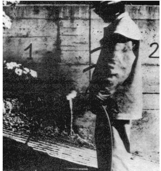
Figure 5-6. Thermal lance
