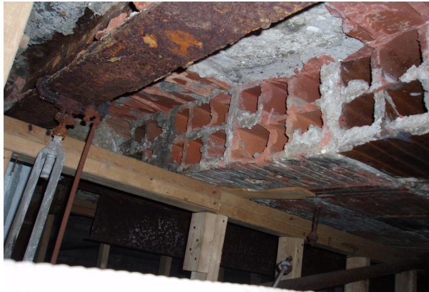
Temporarily Shored Flat Arch End Construction Framing
