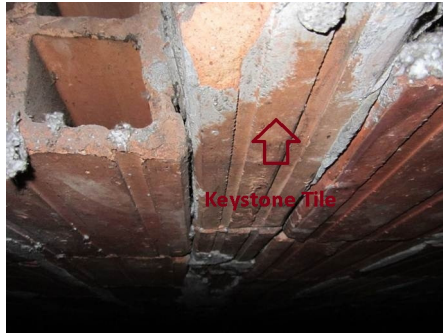
Mid Span Keystone Tile
