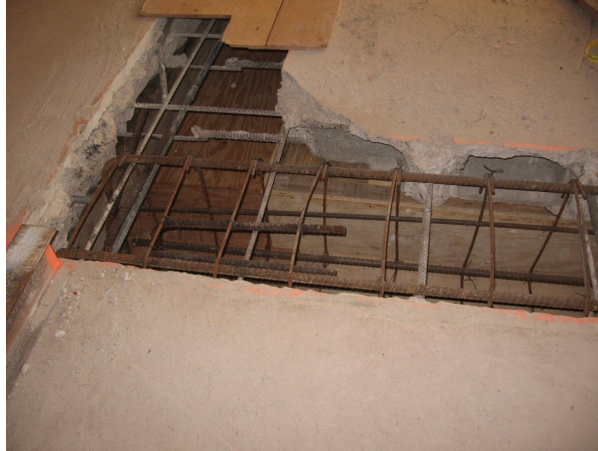
Strengthening of Existing Slab
