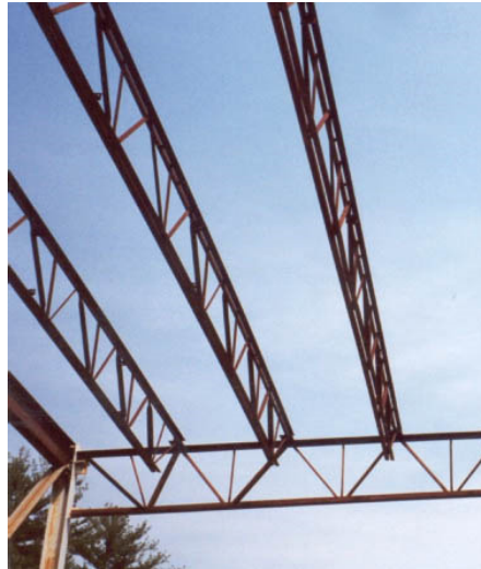
Open Web Joists & Joist Girders
