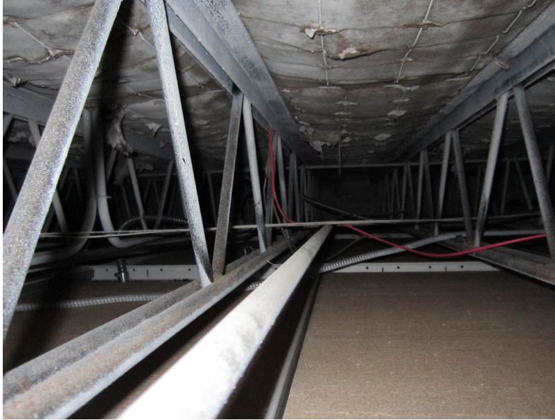
Draped Mesh Slab
