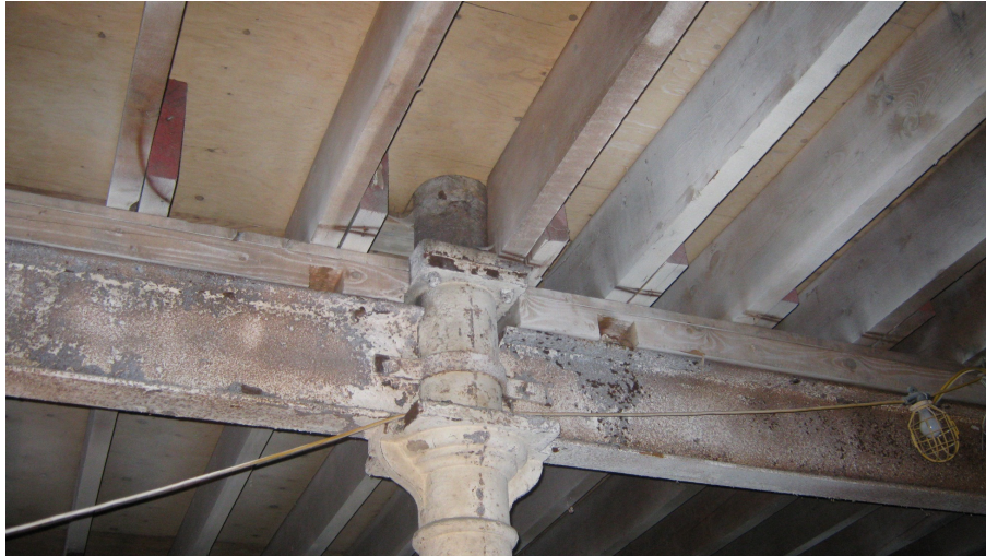
Cast-Iron Column to Wrought Iron Beam Connection
