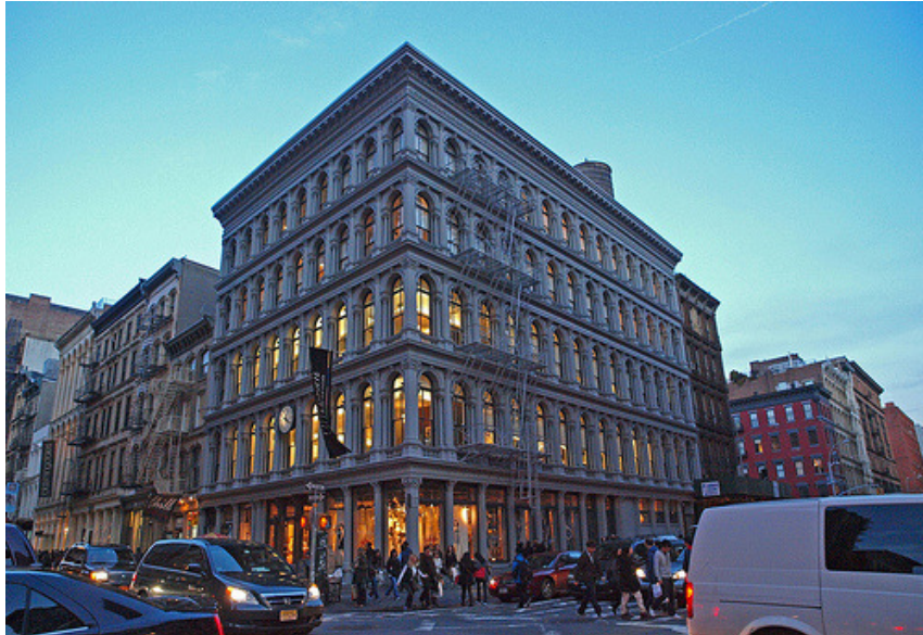
Cast Iron Façade Example E.V. Haughwout Building – New York City Source: Steve Guttman
