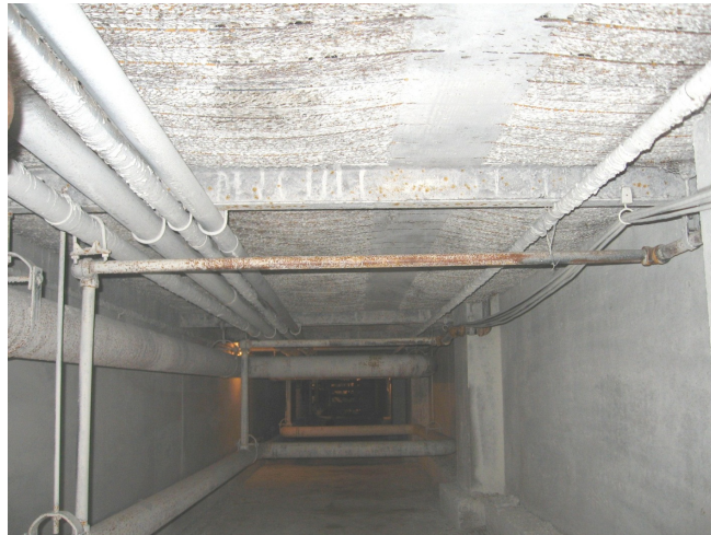
Draped Mesh Slab
