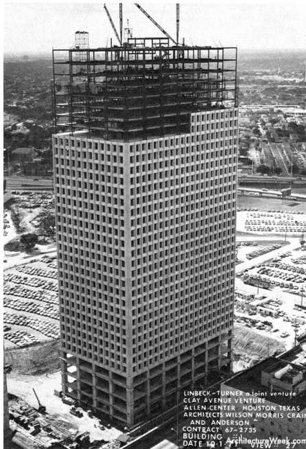
One Allen Center During Construction
