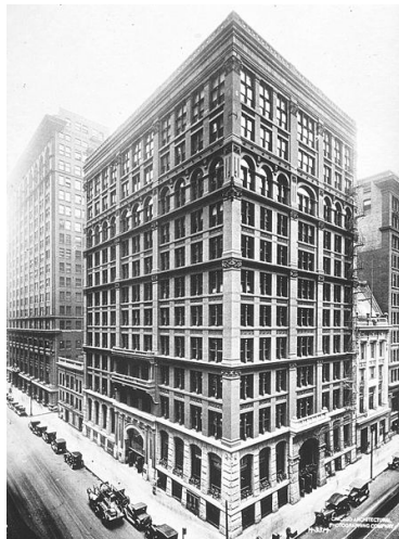
Home Insurance Building Chicago
