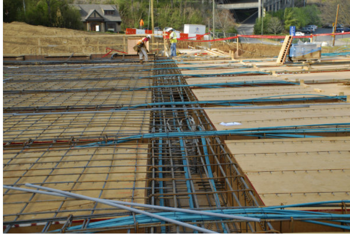
Two-Way Post-Tensioned (PT) Beams
