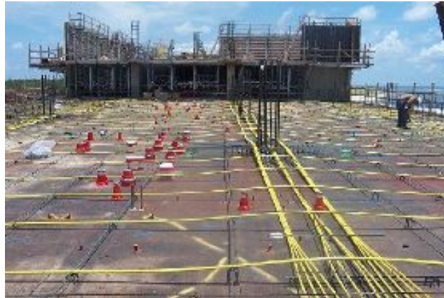
Unbonded Sheathed Post-Tensioning Strands
