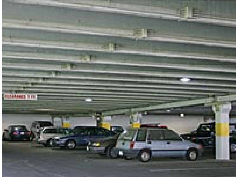
Example of External Post-Tensioning Strengthening
