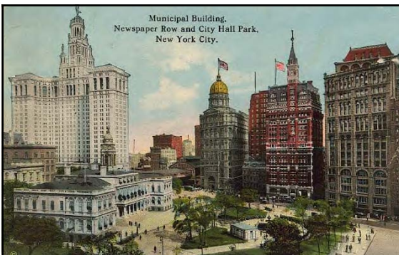
The World Building (at center) was torn down in 1954 to make room for a ramp onto the Brooklyn Bridge
