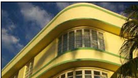
A popular feature of Streamline Deco was the speed line which emphasized the horizontal. Here they serve both as a decorative feature and a functional feature (as awnings to shade the windows from the hot tropical sun). 29
