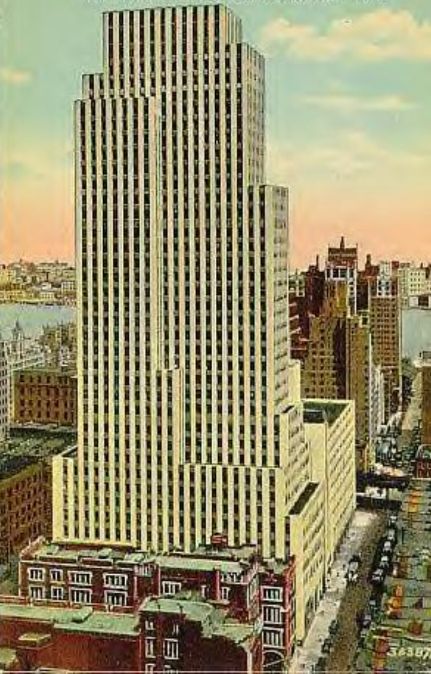
The News Building, 42nd Street, New York.
