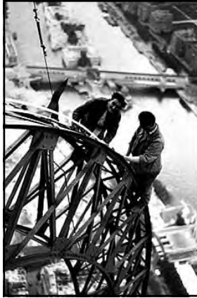
Electricians at Work 1937
