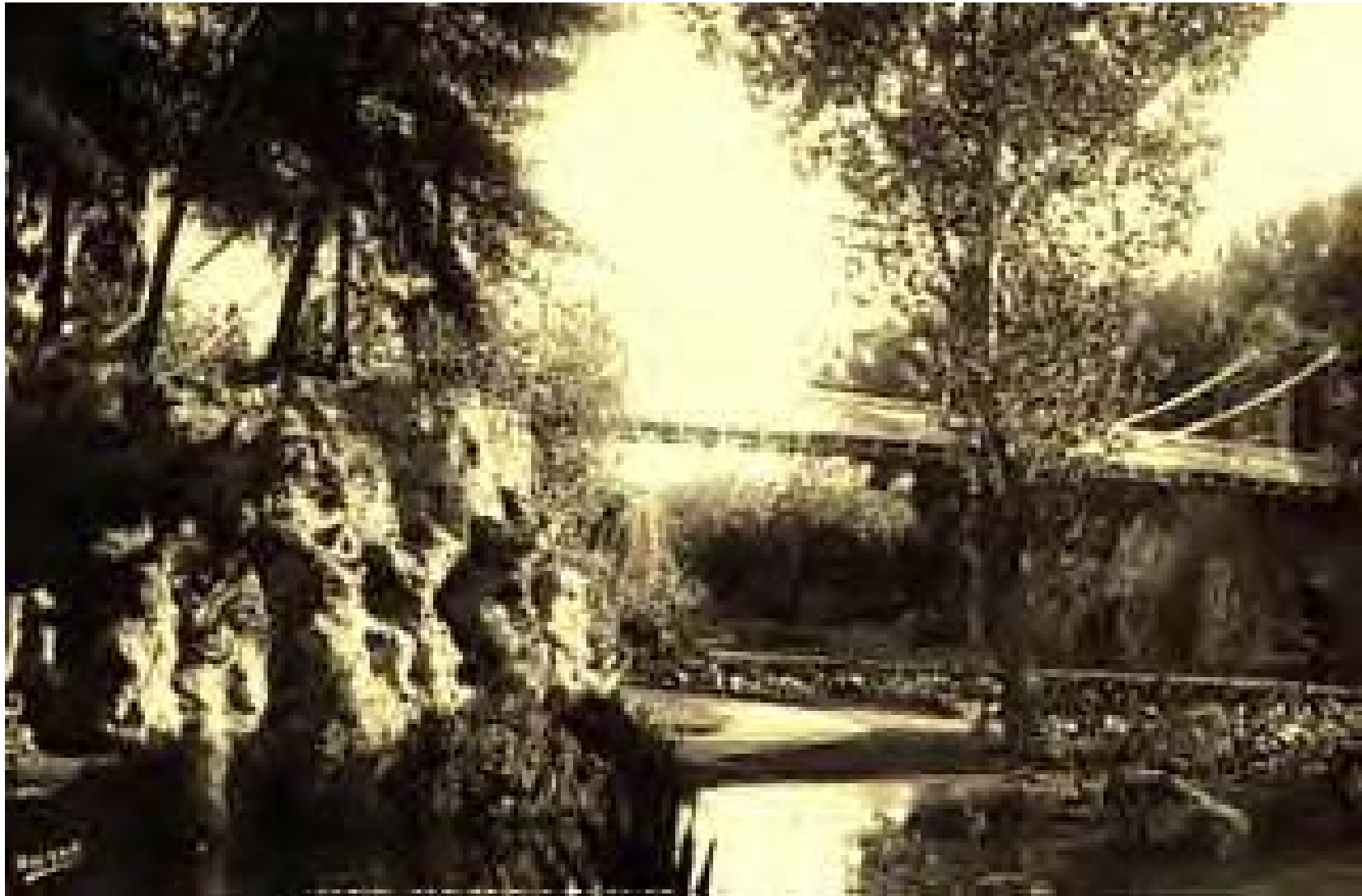
Suspension Bridge Egypt
