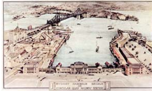
Sydney Harbour Bridge and Circular Quay Railway Station (with cantilever bridge - from Bradfield's doctoral thesis, 1924)
