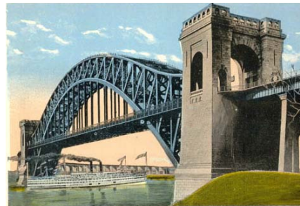
Hell Gate (Railroad) Bridge (1917) New York City (designed by Gustav Lindenthal)
