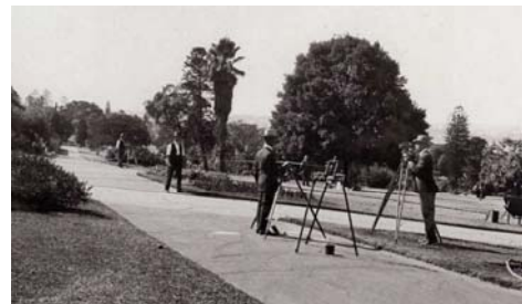
March 17, 1925 Surveyors measuring Base Line "B" (line E-F) (on the Conservatorium grounds)
