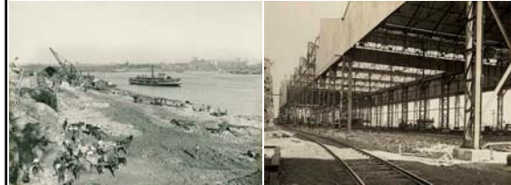
Milsons Point site leveled and cleared (left) Workshops under construction (right)
