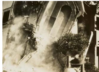
July 1924 Wreckers begin demolishing buildings for the northern approach
