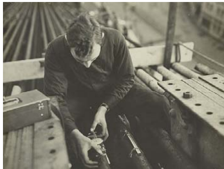
Checking cable tension with pressure gauge 196
