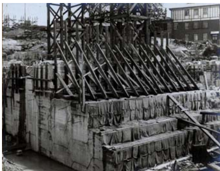
Skewback concrete stepped to receive special concrete (under main hinge-bearing)
