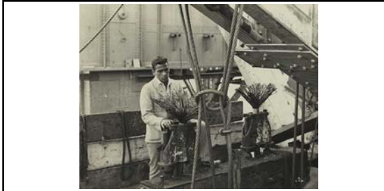
"...To safeguard these vital points, the end of each cable was spread out and secured, by a plug of fused white metal, into a metal socket, this plan providing an attachment equal in strength to the cable itself. These sockets were secured, by equally strong nuts and bolts, in a gigantic steel container, being arranged in eight rows of sixteen..." Wonders of World Engineering, 1938 199
