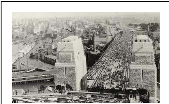
View of South Approach (from top chord of completed arch)
