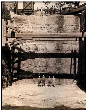
Excavation for the SW Skewback Abutment - April 1926
