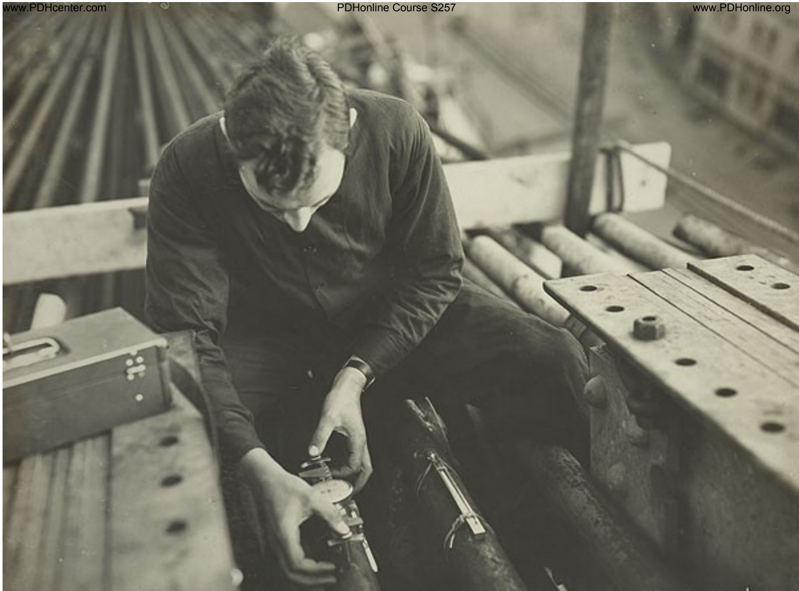
Checking cable tension with pressure gauge 196
