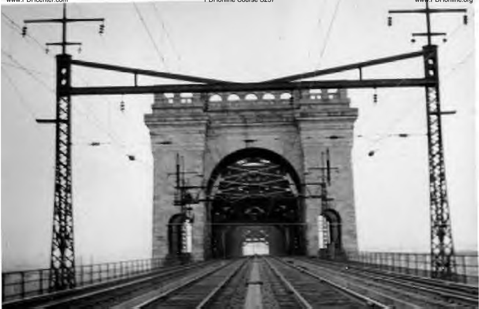
View of pylon, arch and four RR tracks Hell Gate Bridge
