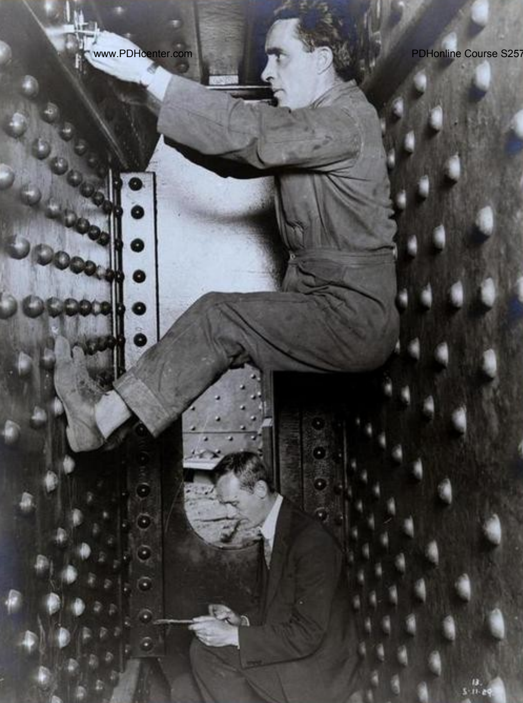
Engineers using strain gauges (within lower-chord)
