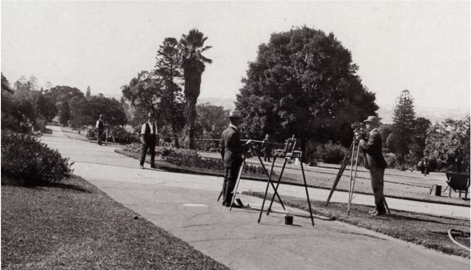
March 17, 1925 Surveyors measuring Base Line “B” (line E-F) (on the Conservatorium grounds)
