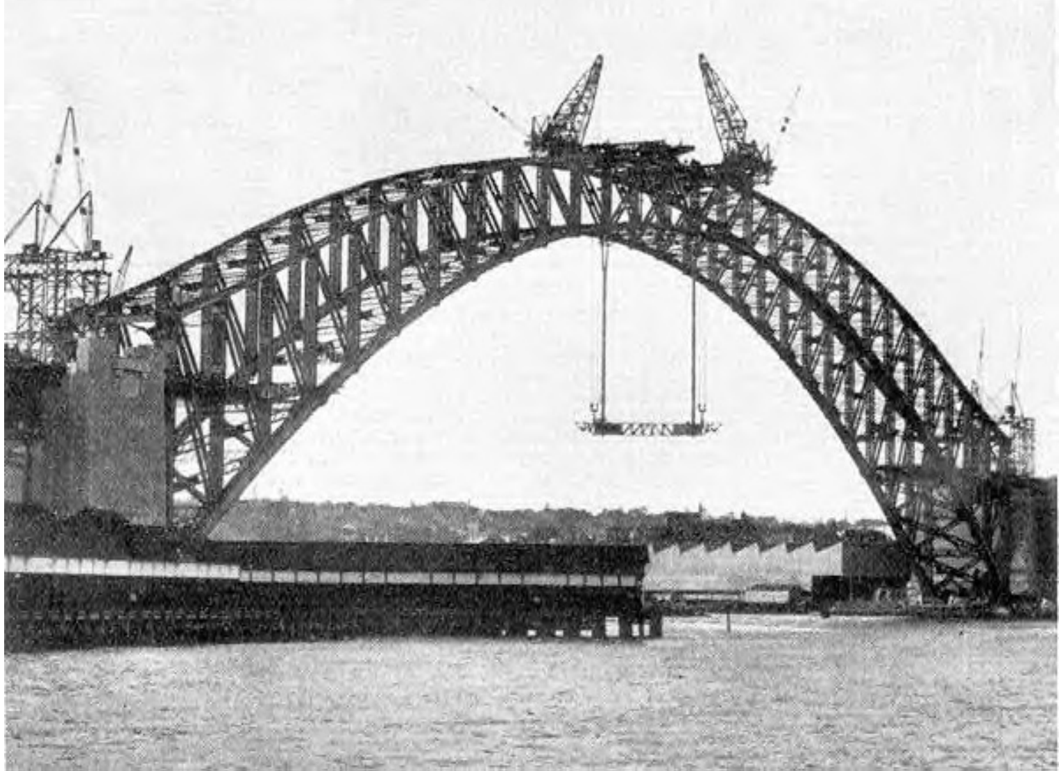
First pair of hangers supporting first cross girder
