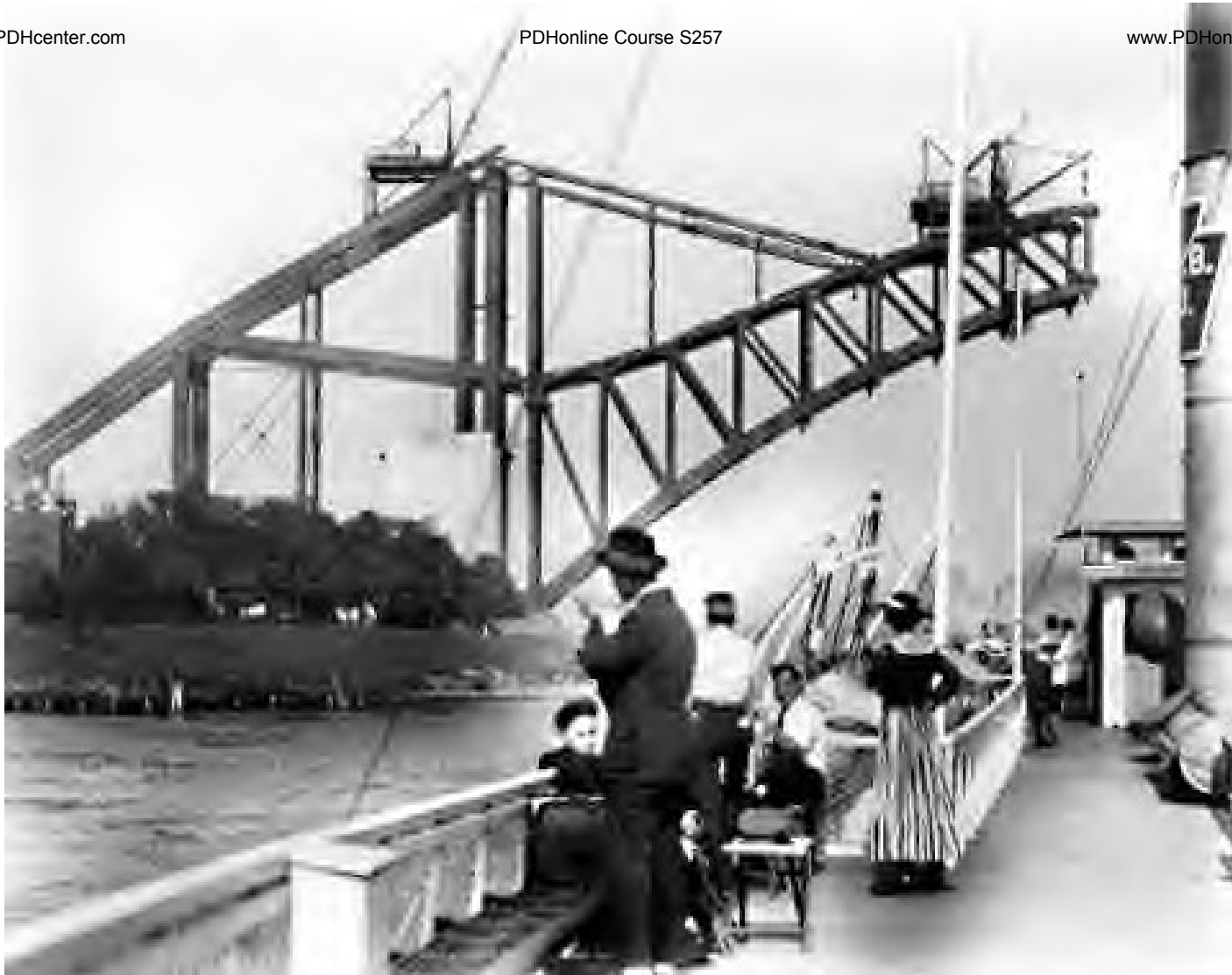
Hell Gate Arch (under construction) ca. 1915
