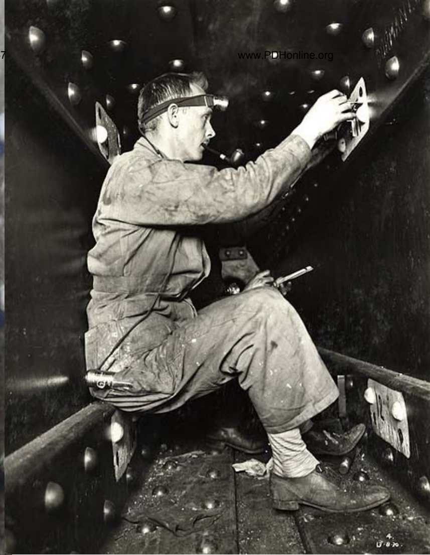
Engineers using strain gauges (within lower-chord)
