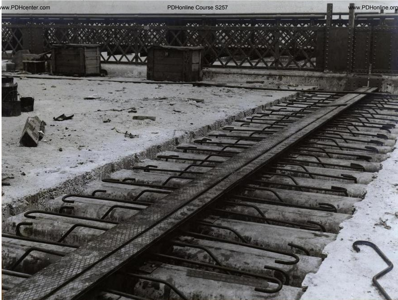
Expansion joint in approach span roadway deck
