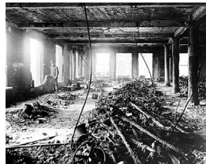
Aftermath of the Triangle Shirt-Waist Factory Fire (the structure was fireproof, but not the contents)
