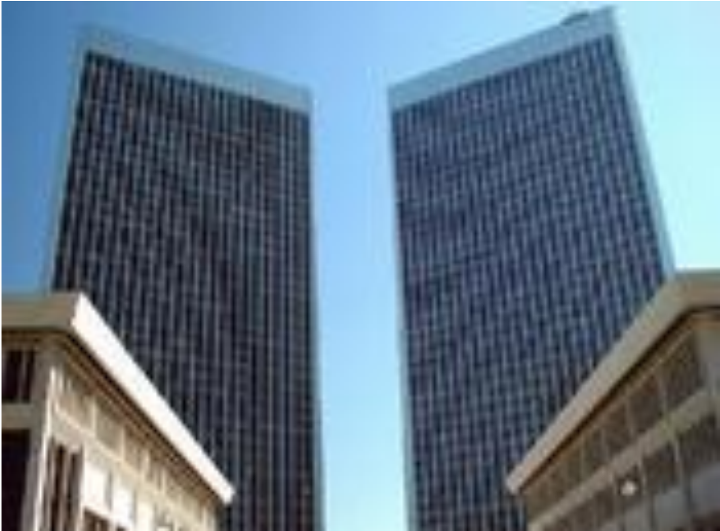
Century Plaza Towers Los Angeles, California
