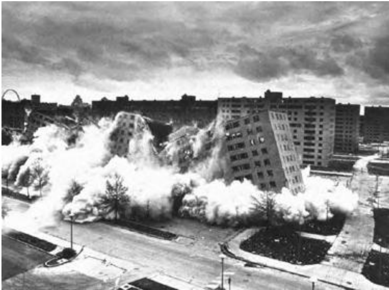
Demolition of the Pruitt-Igoe Housing Project St. Louis, Missouri (July 15, 1972)
