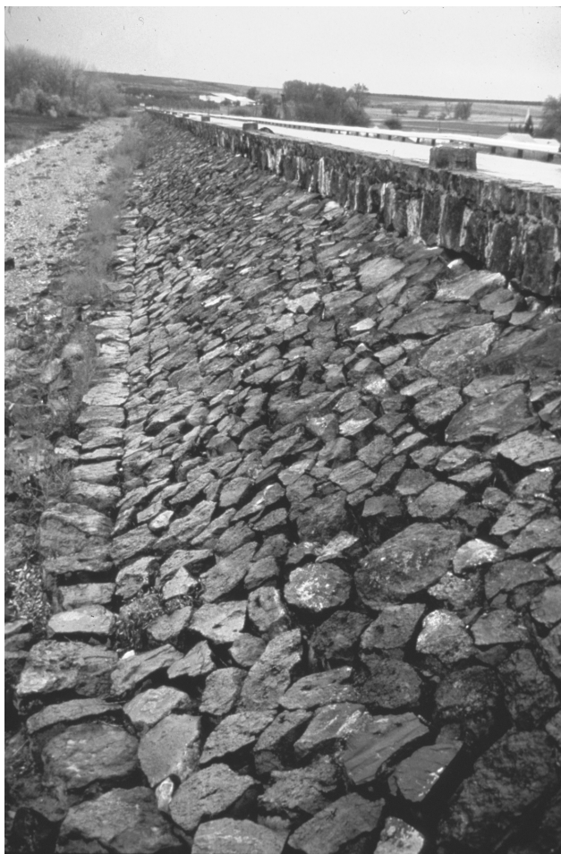
Figure 18-3.—Hand-placed riprap.
