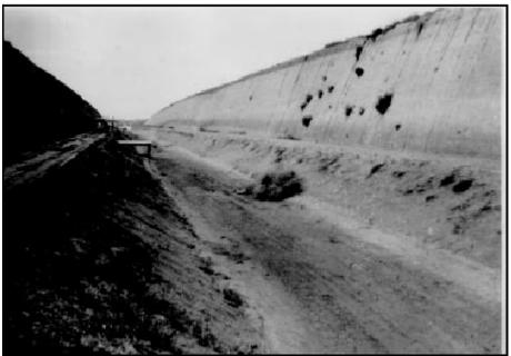
Figure-22.—A 34-foot cut on 1/2:1 slope in loess formation—Franklin Canal, Nebraska.
