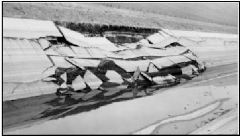
Figure-29.—Slope failure and bottom heaving of Friant-Kern Canal, California.
