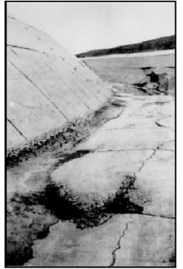
Figure-30.—Heaving of canal bottom (about 300 mm at center), Mohawk Canal, Arizona.
