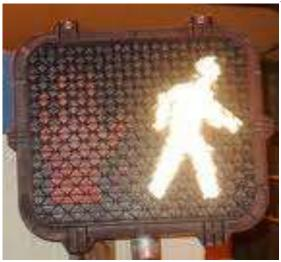
WALK intervals of greater than 7 seconds may be used where the duration of the associated vehicular green interval is long enough to accommodate it. The purpose of the WALK interval is to provide enough time for a group of waiting pedestrians to enter the crosswalk before the flashing DONT WALK commences.
