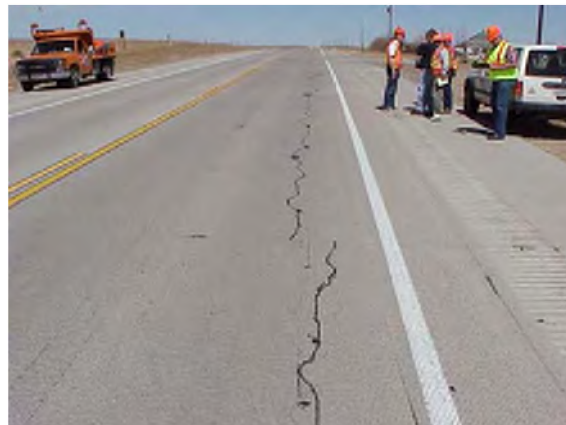
Figure 2. Longitudinal crack
