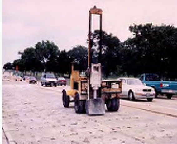
Figure 8. Breakup via drop hammer
