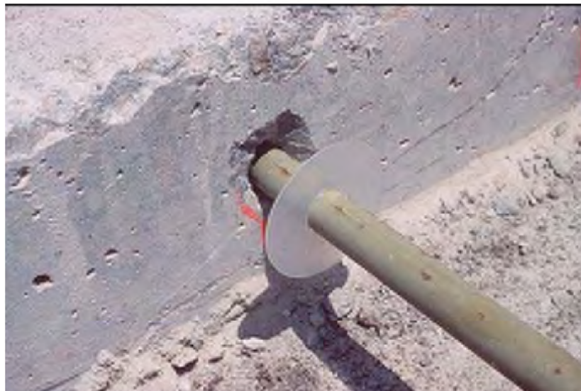
Figure 10. Grout retention disk
