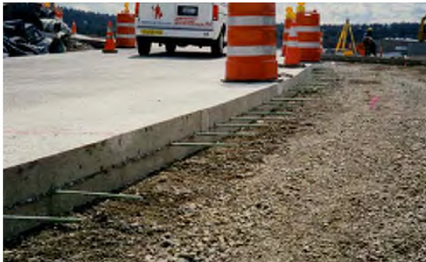
Figure 11. Tie bars along a longitudinal joint
