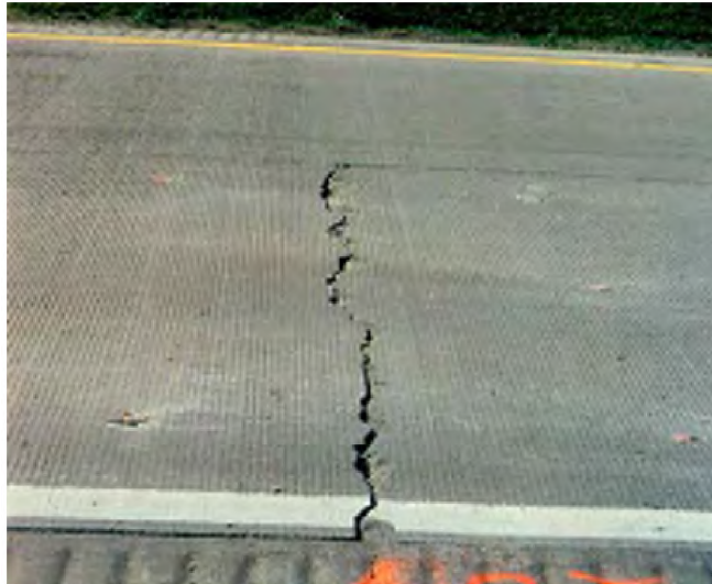
Figure 1. Transverse crack
