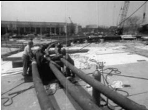
Weighing three-tons each, the orbit rings were field-welded into a continuous single piece, 450-feet around. Special care was taken to protect the polished surface. 257
