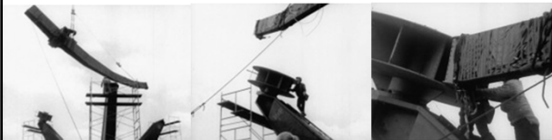
Next, one of Unisphere's largest members, a lower meridian section was fit into the South Pole and laid across the pedestal.
