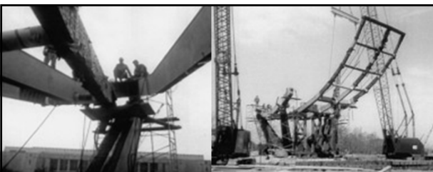
Actually welded girders, the lower meridians support the entire structure. At the site, many of the members were field-welded into sub-assemblies nick-named "orange peel sections."
