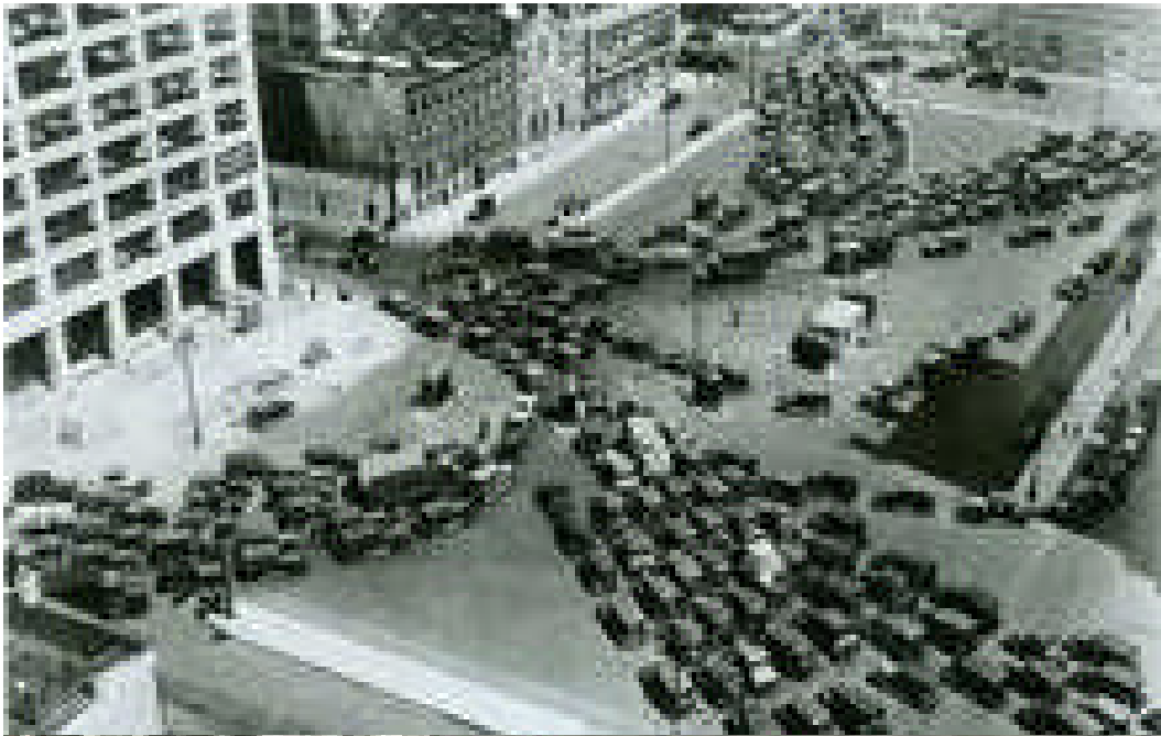
Top: caption: “Holland Tunnel entrances in New York City, 1929”
