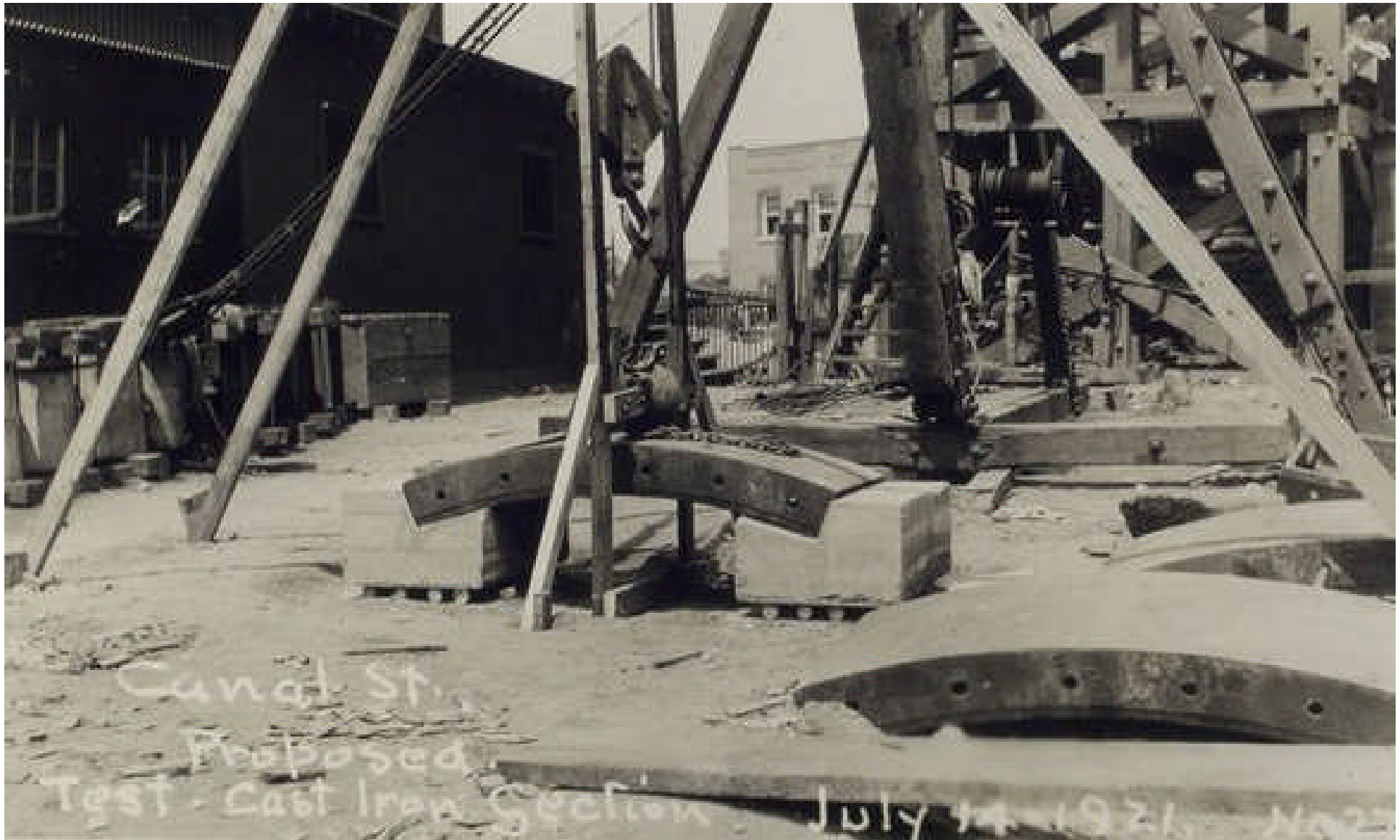
Above : caption: "Proposed test - Cast Iron section. Canal Street, July 14, 1921."
