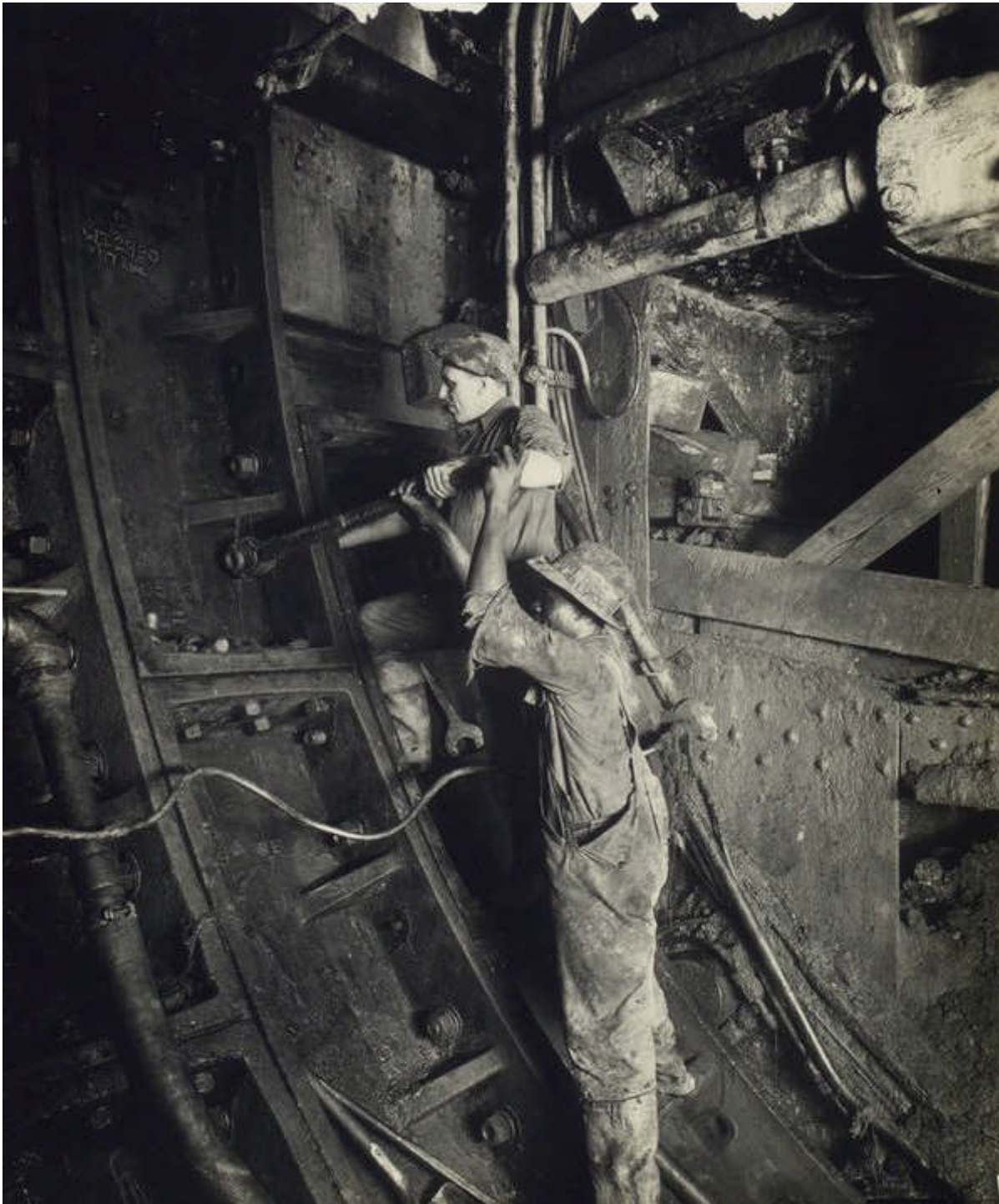
Above Top: caption: “Steel pile segments and forms for setting concrete invert. 4/30/25.”
