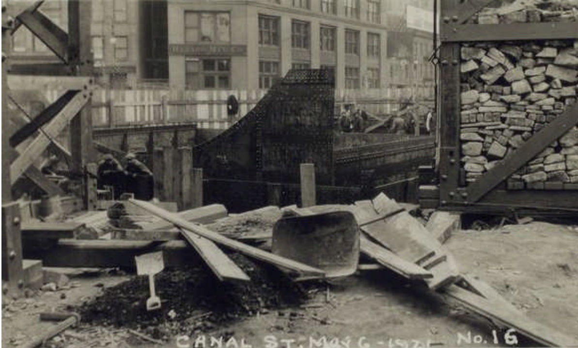
Bottom: caption: “West side, inner and outer skin plates. Canal Street, May 6, 1921”
