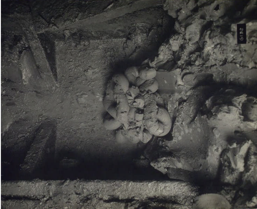
Top Left: caption: “Cleaning, caulking, pointing and making iron watertight invert, South Tunnel east, N.J. 12/5/24.”
