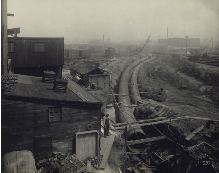
Top Left : caption: “Completed portion 5’ steel sewer, Jersey City, N.J. 5/21/25.”
