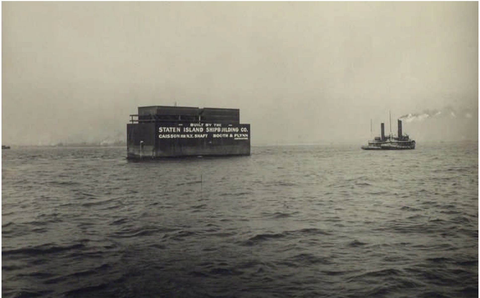
Above: caption: "General view New York River Shaft Caisson. Upper New York Bay North of St. George, S.I. 1/20/23."
