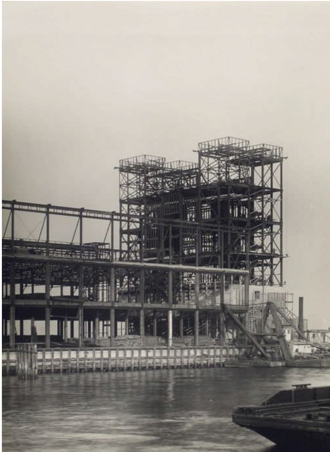
Left: caption: “Steel framing - River Ventilation Building, New Jersey. 11/22/26.”
