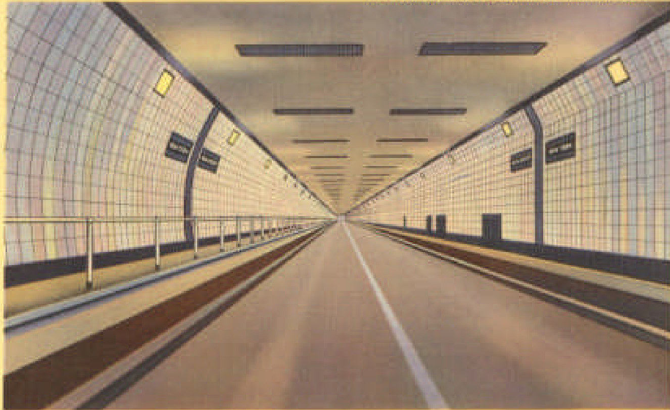
INTERIOR OF HOLLAND TUNNEL, NEW YORK CITY
