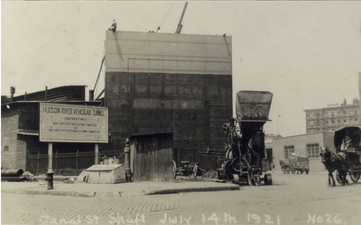
Bottom: caption: “Pai- nting. Canal Street Shaft, July 14, 1921”
