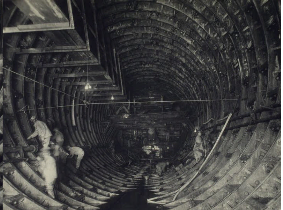
Top Left: caption: “Cleaning, caulking, pointing and making iron watertight invert, South Tunnel east, N.J. 12/5/24.”
