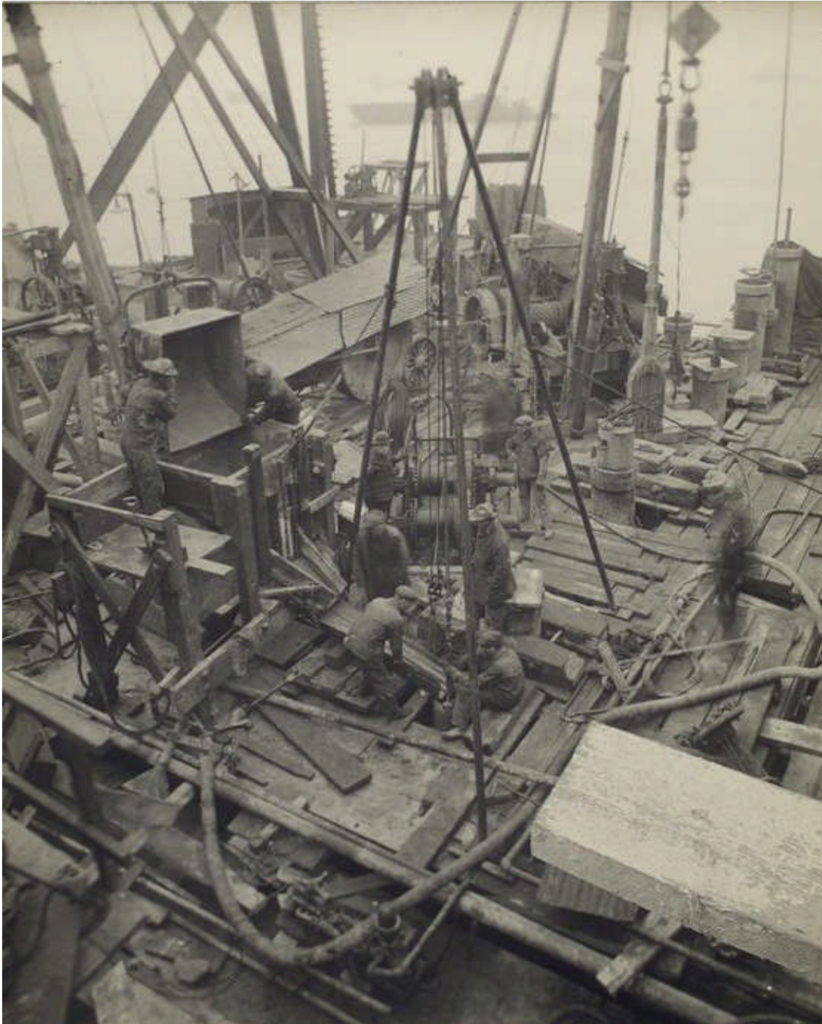
Left: caption: “Reinforced Concrete piles, South River shaft. New Jersey. 5/15/23.”
