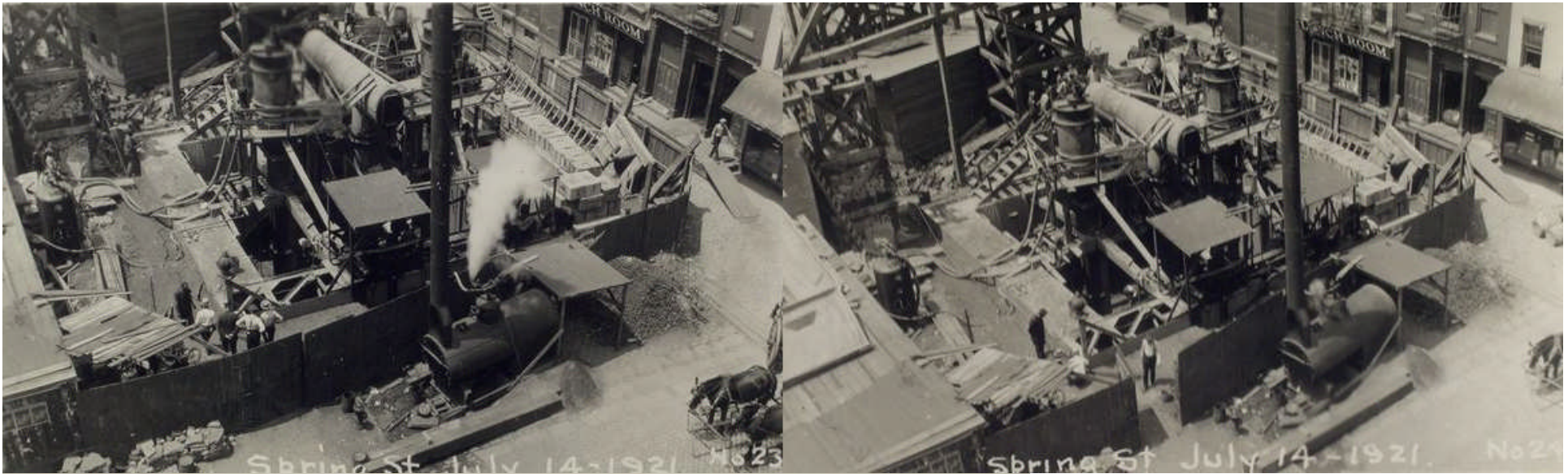
Top Left: caption: “Cai- sson top about 16 inches above surface. Cast iron weights N.E. corner. Slight fissures showing at left side. Spring Street, July 14, 1921.”
