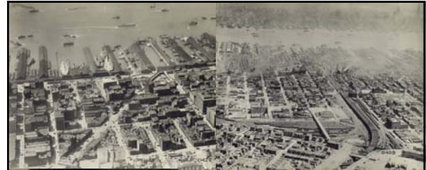
Top Left: caption: "Aerial photograph of tunnel site in New York, looking West. 5/4/23" Top Right: caption: "Far view of New Jersey approach. 7/28/23" Left: caption: "Nos. 248-250 Erie Street being removed from exit plaza, Jersey City, NJ, 5/24/26" 452
