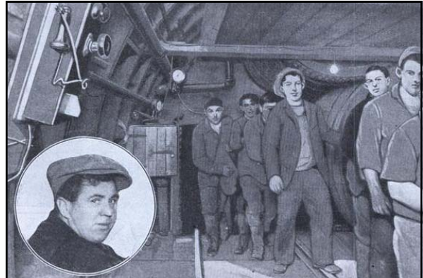
Above: caption: "Extreme air pressure allows tunnel builders to work only about one hour in five. A crew is shown coming off duty to rest five hours before re-entering the tunnel. Insert shows Walter Redwood, whose career is told in this story." 572
