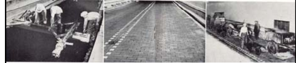
Above Left-to-Right: caption: "Striking off asphaltic-sand mastic bed course with screed traveling on rollers and discs with compensating carriage / Close-up view of completed brick pavement showing clean wire-cut skid-resistant traffic surface / Kerosene fueled heating kettles in which 'blended' asphalt filler was heated to 450-degrees F"
