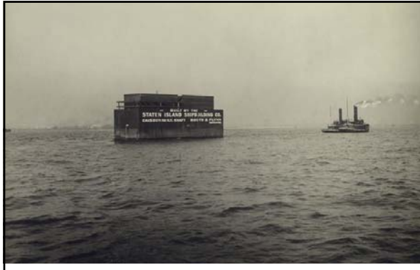
Above: caption: "General view New York River Shaft Caisson. Upper New York Bay North of St. George, S.I. 1/20/23." 547
