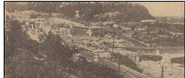
Above: caption: "Just as time marches on, so does construction work on the Weehawken Midtown Tunnel. Here is a view taken of the latest advancements made on the approaches. No. 1 shows the mouth of the tube crossing from the western to the eastern side of the Hudson River. No. 2 is Park av., widened. No. 3 is the first completed section of the overpass crossing Boulevard East. The pass will be built farther south and will circle back north alongside King's Bluff and west into Union City. The stretch of dirt road in the foreground is Hackensack av., better known as the 'High Road,' which will also be rebuilt. No. 4 is the administration building now in process of construction. This will house the business department of the Port of New York Authority who will concentrate on tunnel work. No. 5 is where the overpass will circle around and back into Union City. Workmen are busy constructing concrete pylons and blasting away the rock hills just north of the town." (Hudson Dispatch, August 19th 1937) 874
