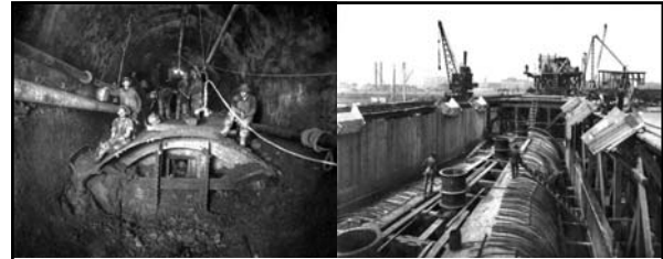
Left: caption: "View east in the old south tunnel not far from the 15th Street shaft, 1905. The shield is moving toward the camera and down, to establish the new lower level approaching the junction just west of the 15th Street shaft. This shows the tall elliptical shape of the oldest portions of tunnel."
