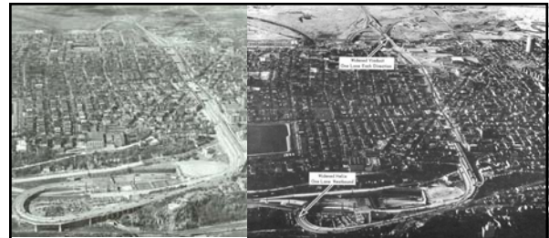
Left: caption: "New Jersey Approaches prior to start of construction of the Third Tube Project" 940 Right: caption: "New Jersey Approaches after completion of the Third Tube Project"
