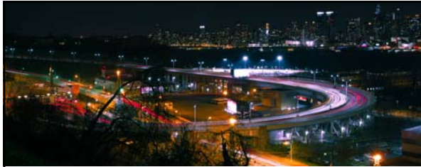
Above: caption: "That great curving ramp, called a helix by the engineers who built it, leads down into three of the world's most expensive holes in the ground: The triple-tube Lincoln Tunnel from New Jersey to New York City. Eighteen traffic lanes pass under the toll booths on the plaza at lower left, and they merge into six as they enter the tunnel. Beyond the Hudson River, the lights of the metropolis glamorize the night. The tallest building (upper left) is the Empire State. Each day, nearly 40,000 automobiles go underground here at Weehawken, N.J. and emerge after a five minute trip on the west side of Manhattan between 38th and 39th Streets. And an equal number escape the jammed streets of the crowded island and sweep back up the helix. The impatient drivers take little note of the design which their headlights emphasize, but they are part of an accidental pattern of beauty. And even these weary travelers must find subconscious satisfaction in traversing this mighty spiral, upward and outward from deep beneath the river." 937 Saturday Evening Post, September 1958
