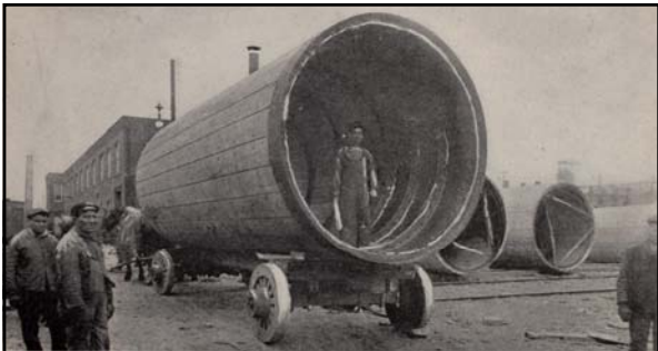
Above: caption: "One of the mammoth caissons about to depart for fields of useful engineering endeavor"
