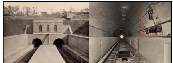
"...The through trains to New York leave Harrison on rails crossing over the old Pennsylvania tracks on a steel and concrete bridge. A double-track elevated line on embankments and bridges extends across the Hackensack Meadows to Bergen Hill, that high eminence which is a continuation of the rocky cliffs extending along the Hudson River. In the western slope of this hill are found the entrances to the tunnels which lead under the North River, into the Station in New York..."
