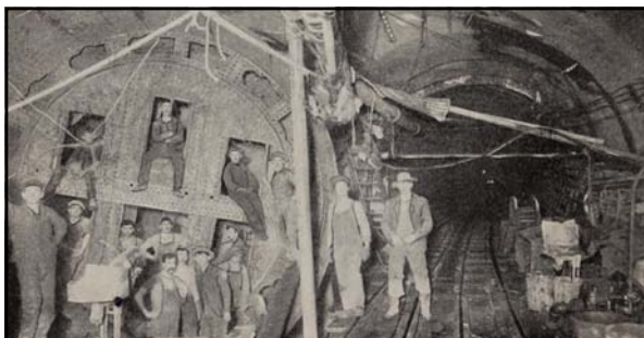
Above: caption: "Having arrived at the terminal, here we see another shield (at left) about to begin its mission for the betterment of transit facilities between the two states" 161
