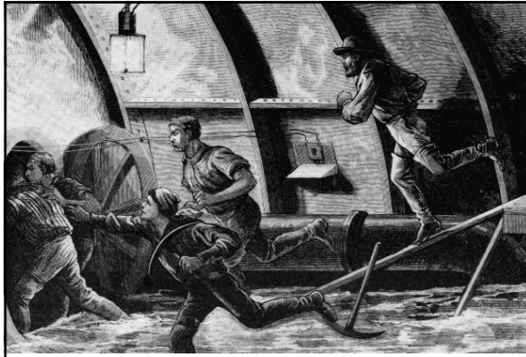
Above: caption: "Artist's conception of miners escaping into the air lock during the blowout in Haskin's tunnel" 109
