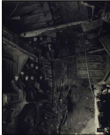
Left: caption: "North Tunnel - New York and New Jersey shields the day prior to their junction"
