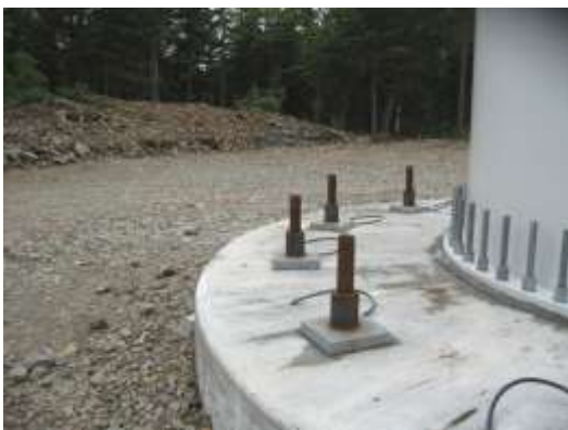
Portion of foundation, and structure grounding for a 3 MW wind turbine
