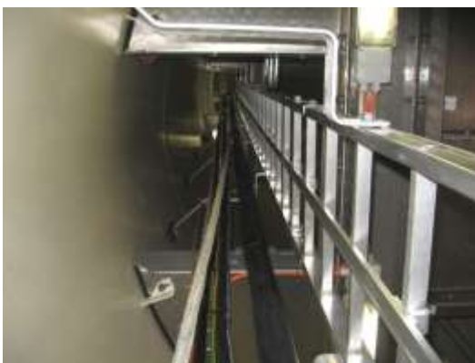
View of climbing tower inside a 3 MW wind turbine structure
