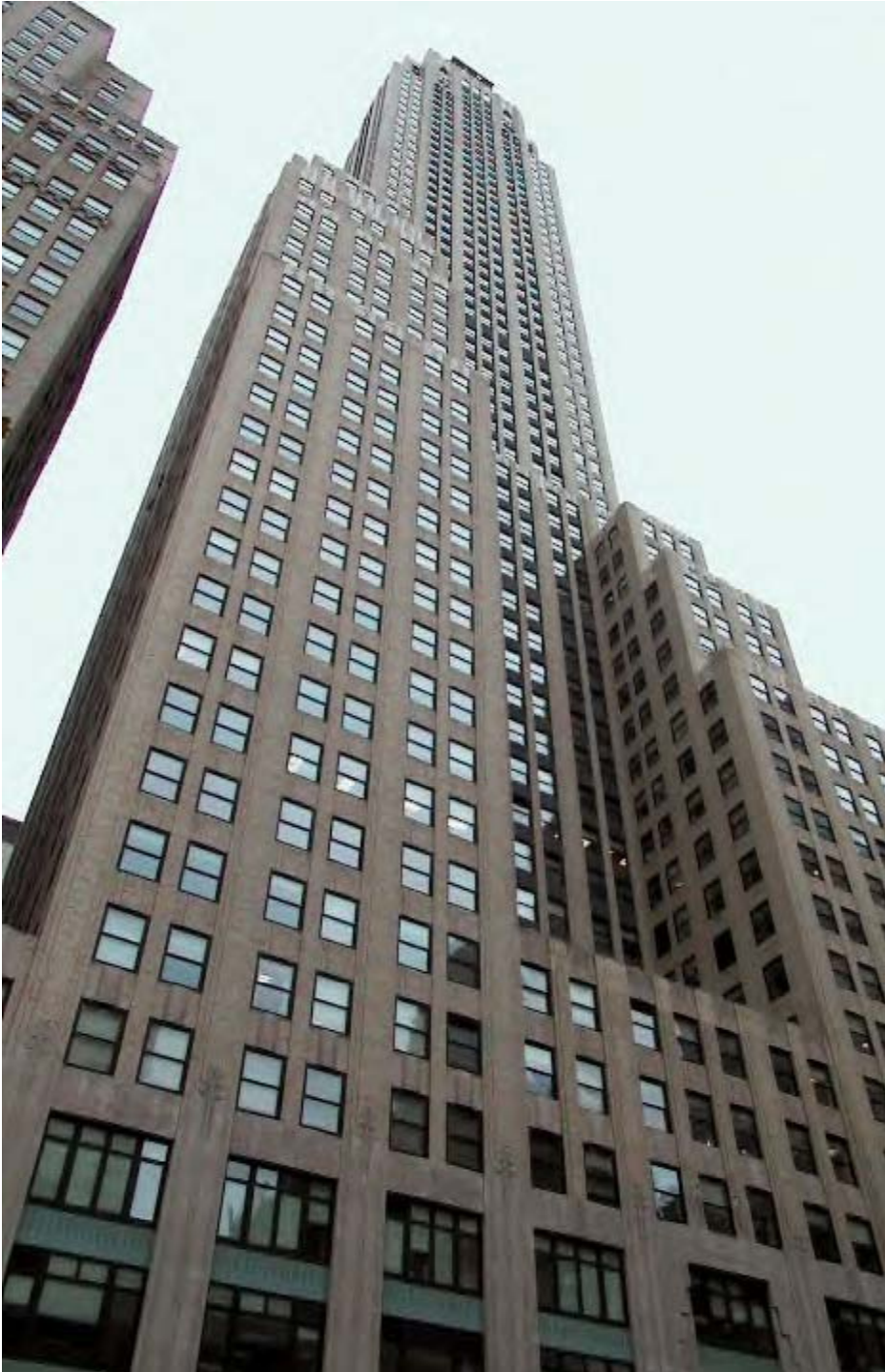
500 Fifth Avenue Shreve, Lamb & Harmon, Architects, 1929 (design forerunner of the Empire State Building)
