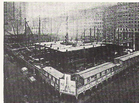
FIG. 2—EARLY ERECTION VIEW OF EMPIRE STATE BUILDING
