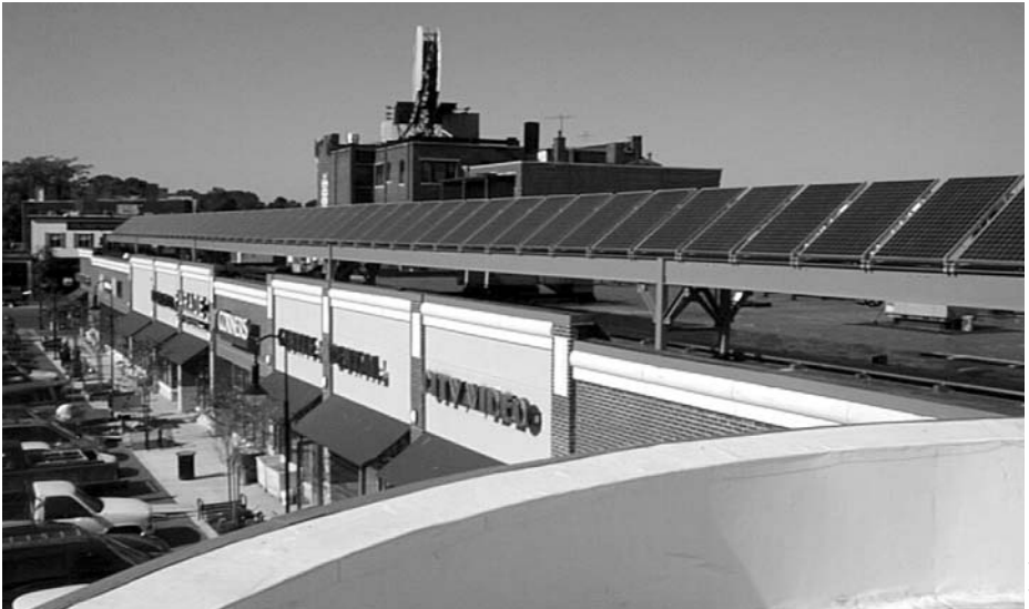
This 20-kilowatt PV system produces electricity for the common areas of a shopping center in Cambridge, Massachusetts.
