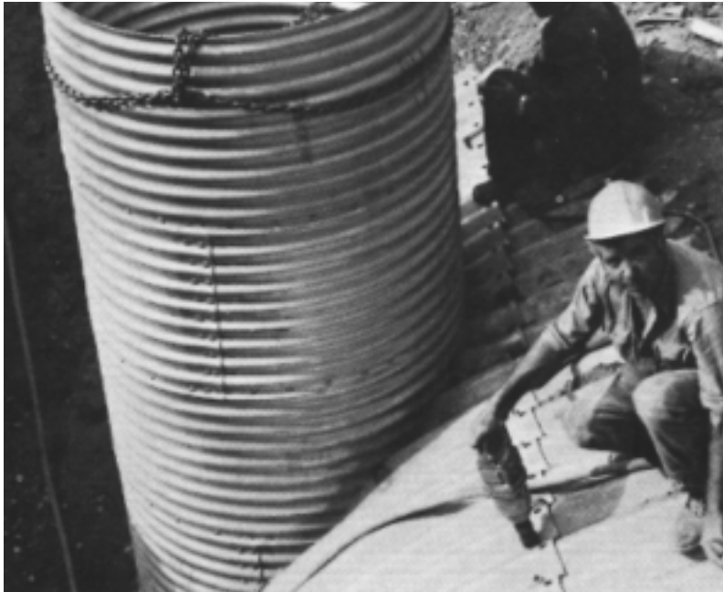
Joining factory made CSP into large structural plate storm drain.
